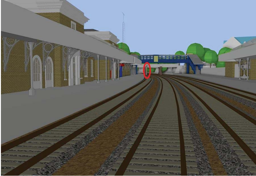
Signal NK438 could be sighted under the new footbridge
