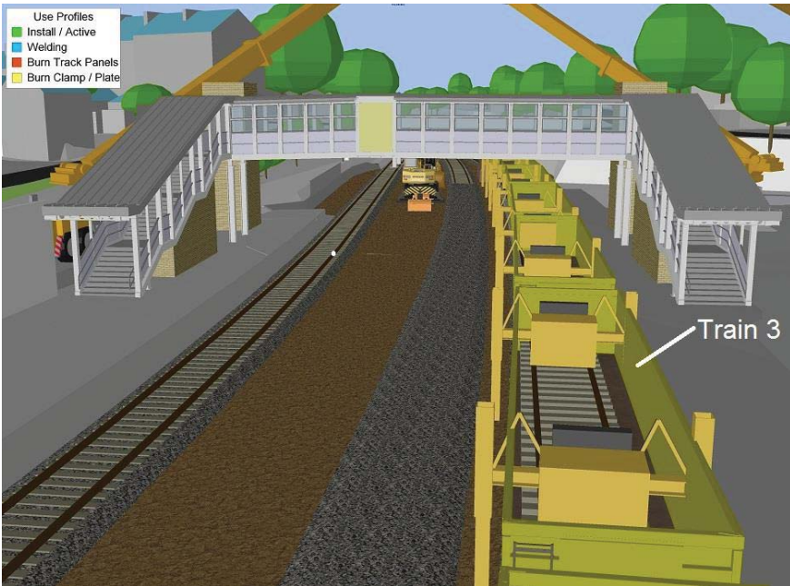
2. Track to be repositioned using PEMs clashes with an engineering train.
