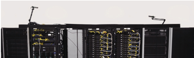
Fig. 3. The prototype of mmWave radios are equipped on the racks in cloud center.
