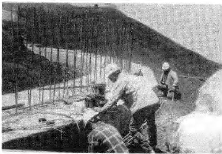
Constructing the base for the Keck I dome. (Courtesy Keck Observatory)
