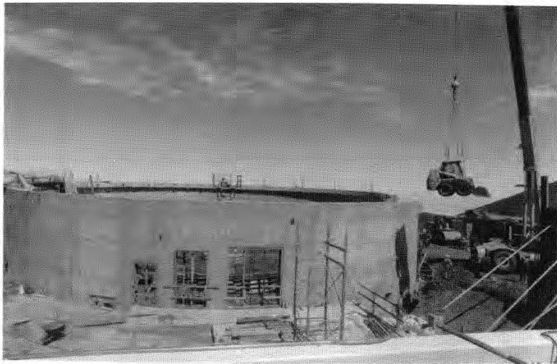
Building the Keck II dome.
