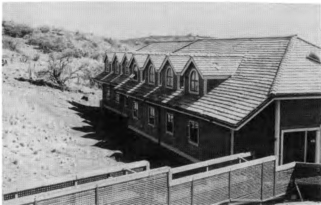
View of the sleeping quarters from the dining hall at Hale Pohaku.
