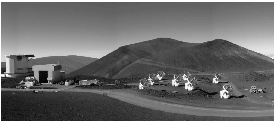
Fig. 1. The Submillimeter Array near the summit of Mauna Kea in its nominal compact configuration, similar to the one used for the observations described here. The vehicle on the right is the antenna transporter, which is used to move the antennas among various configurations. The cylindrical dome on the left is the James Clerk Maxwell Telescope, which will be included as an element in the SMA, along with the CSO, later in 2006.
