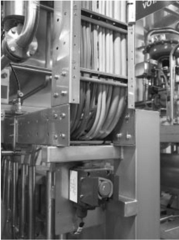
Fig. 15.3 Cables beside each other on a stainless steel cable ladder. Note the closed supports and cleanable conduits. Problem: the horizontal parts and omega rail of the cable ladder!
