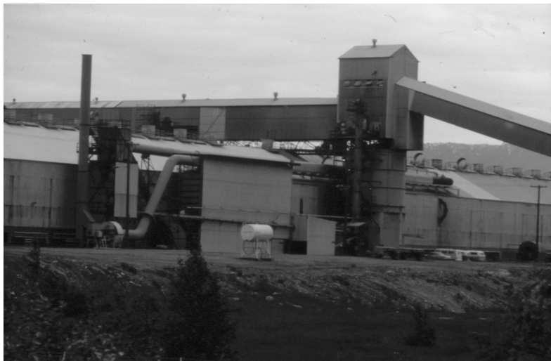
Close-up of the pneumatic conveying facilities used in the operation of the dry scrubber for plant-wide control and recycling of volatile fluorides.
