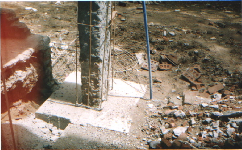
Figure 4: New pad foundations.
