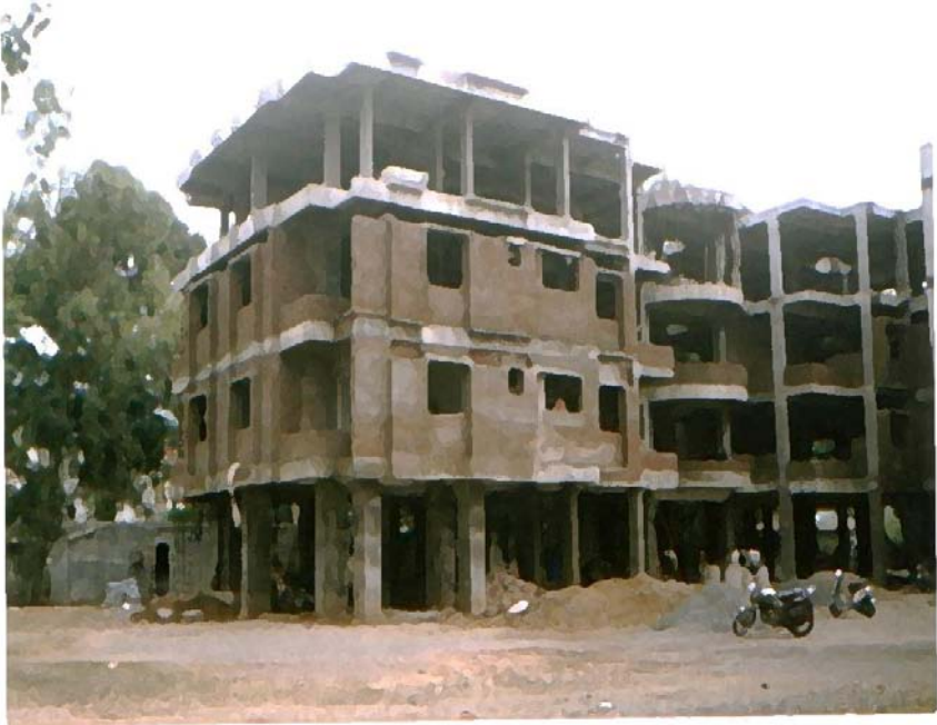
Figure 2: Photo of the building being constructed.
