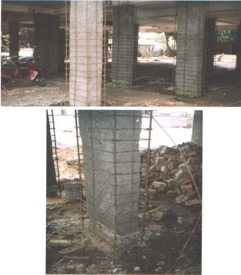
Figure 3: Jacketing of columns.
