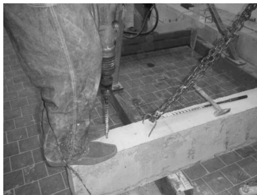
Figure 2. Drilling of holes for specimen IER.
