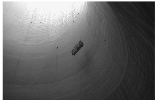
Figure 14. View of all areas with finished coating.
