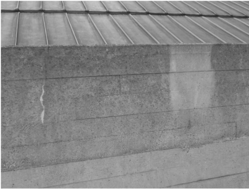
Figure 3. Result of graffiti removal.
