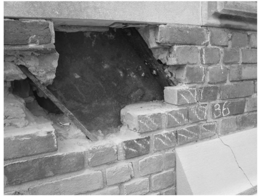
Figure 6. Gable end detail. Note corrosion scale within web and cracking stemming from flange.
