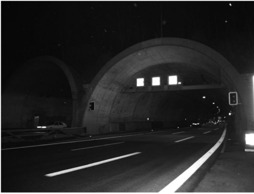
Figure 10. View on the tunnel entrance.
