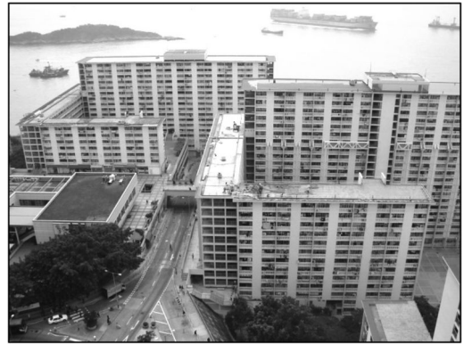
Figure 3. General view of 40-year-old PRH buildings.
