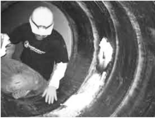
Figure 6(a). Installation of FRP in pipe.
