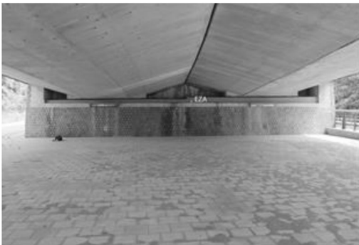
Figure 7. EZA installed on the beams supporting the bearings of the Hubertus viaduct in The Hague.
