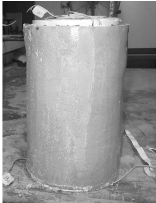
Figure 2. Specimen after ferrocement jacketing.
