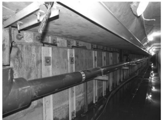
Figure 7. Cassette system installed in confined space.
