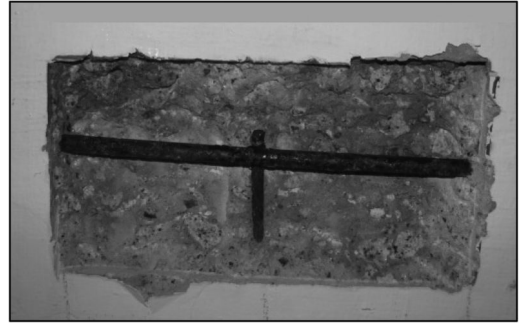
Figure 7. Concrete breakout for inspection of corroded steel reinforcement.
