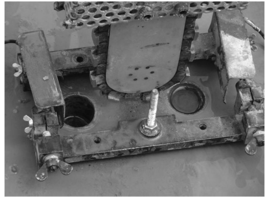
Figure 3. Measurement frame and core holes prior to forming the slot.
