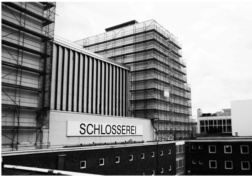
Figure 2. Construction site of the Cologne Opera.
