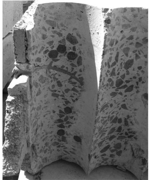
Figure 7. Block removed from infill slab showing concrete intrusion into movement joint above and below waterstop.
