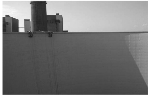
Figure 13. Finished coating of upper third to the right of the picture.
