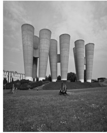
Figure 3. Example of group of adjacent elevated tanks.
