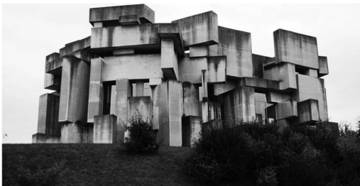
Figure 1. Wotruba Church. View from north-east side.
