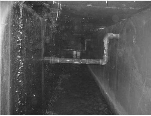
Figure 2. Environment within a wet duct environment.
