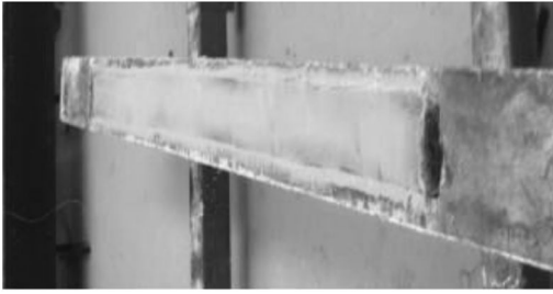
Figure 3b. Beams before grouting the beam.
