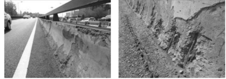
(b) Reinforced concrete crash barrier walls on An Fa Bridge (1990)
