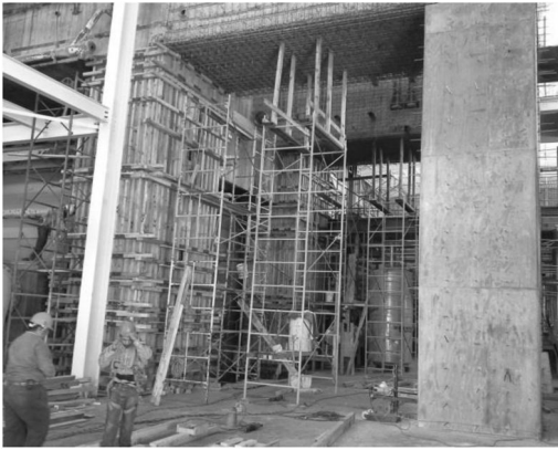
Figure 10. Forming on column, propping, and view of a repaired column.
