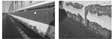
(c) Matsuura Bridge(2010)
