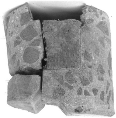
Figure 5. Example of concrete intrusion below filler board and above waterstop.
