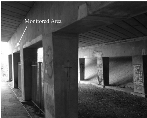
Photo 1. Leicester Bridge abutments with monitored area indicated.
