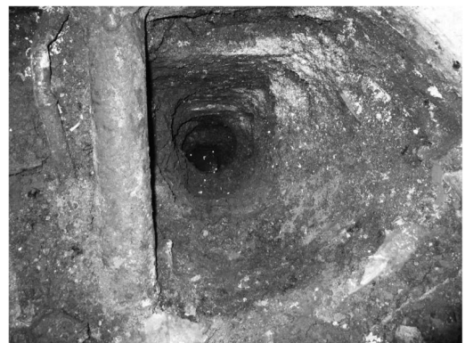
Figure 4. Foundation examination pit.
