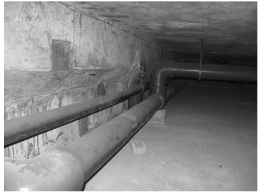
Figure 3. Access difficulties in dry duct crawl space.
