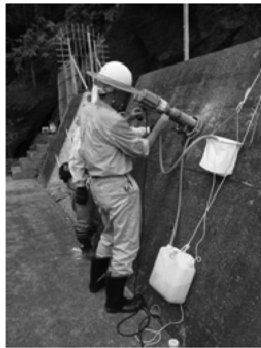
Figure 1. Situation of cutting of the core.
