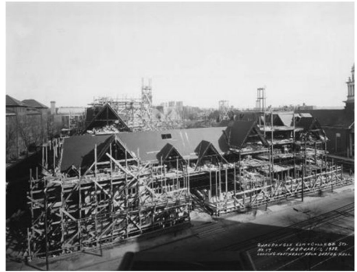
Figure 4. Construction of Calhoun College. Ca. 1931.
