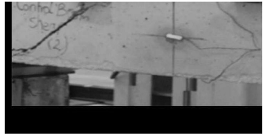
Figure 12. Shear failure for control specimen examined by (Obaidat, 2007).
