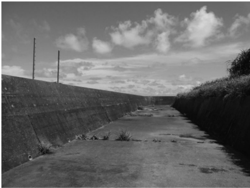
Figure 5. Seawall in outlet of structure B.
