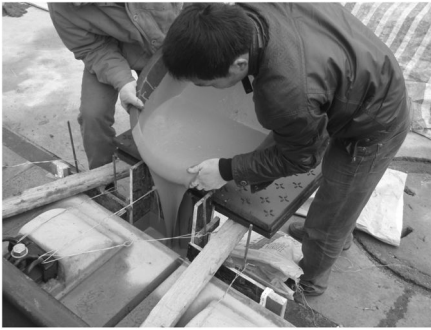
Figure 9. Pouring of polymer modified mortar.
