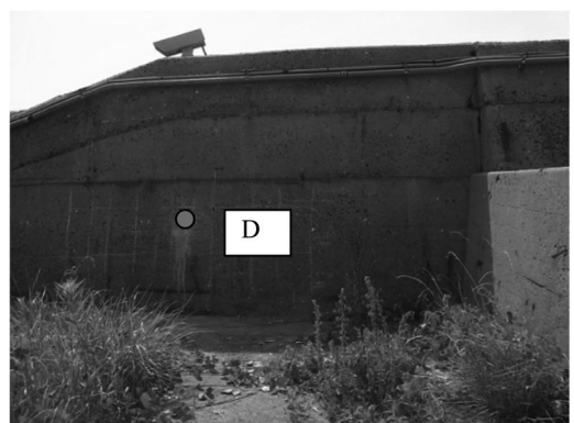
Figure 9. Seawall in intake of structure D.
