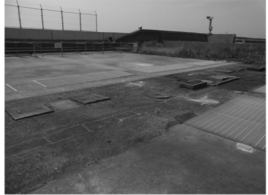
Figure 8. Intake of structure D.
