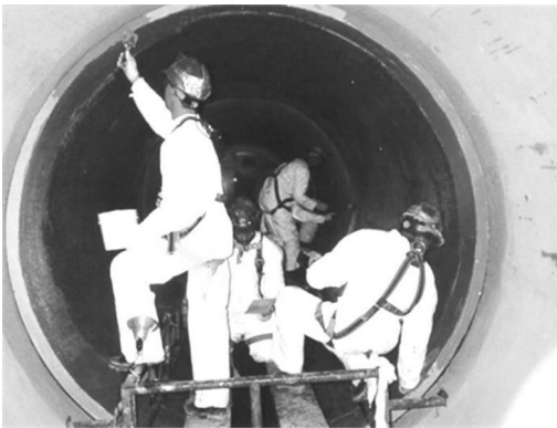
Figure 6(b). Installation of FRP in pipe.
