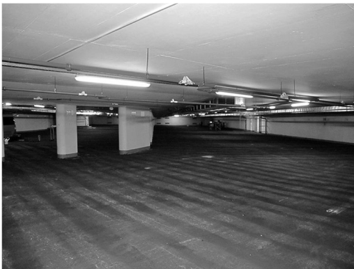
Figure 16. View on the car park after removal of the asphalt layer.
