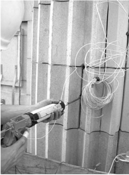
Figure 2. Anode Installation at a Pilaster Column. Author's Photograph.
