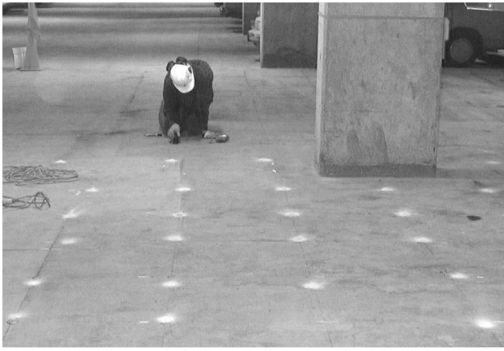
Photo 3. Placing of cylindrical anodes in a grid configuration.
