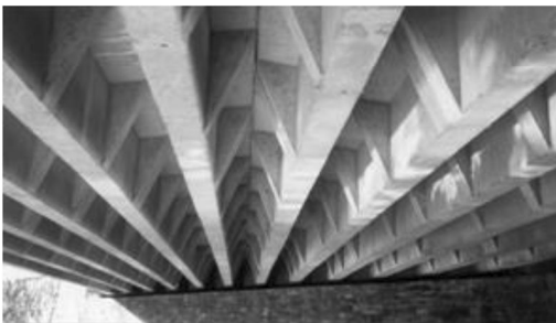
Figure 2. 50 year old segmental bridge in excellent condition.
