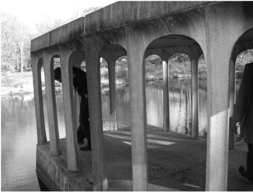
Figure 5. Pavilion on the Pond. Authors photograph.
