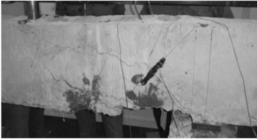
Figure 9. Crack patterns of specimen S-IER.
