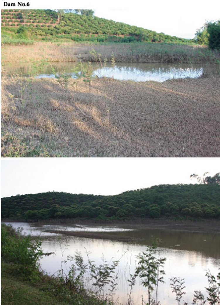
Fig. 29.5 Inability to store design water capacity because of leakage
