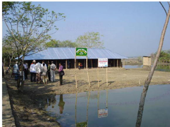
Fig. 15.8 Partially damaged school ( Source Save the Children, 2010)
