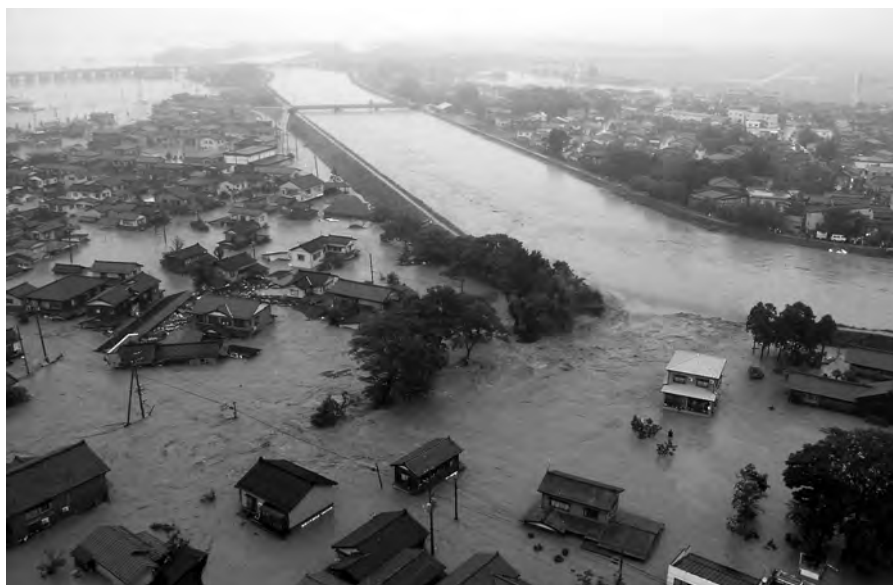
Photo 2. Flood water flowing into the housing area from the bank break site of Kariyata River (Photo by Kyodo-Tushinsha).
