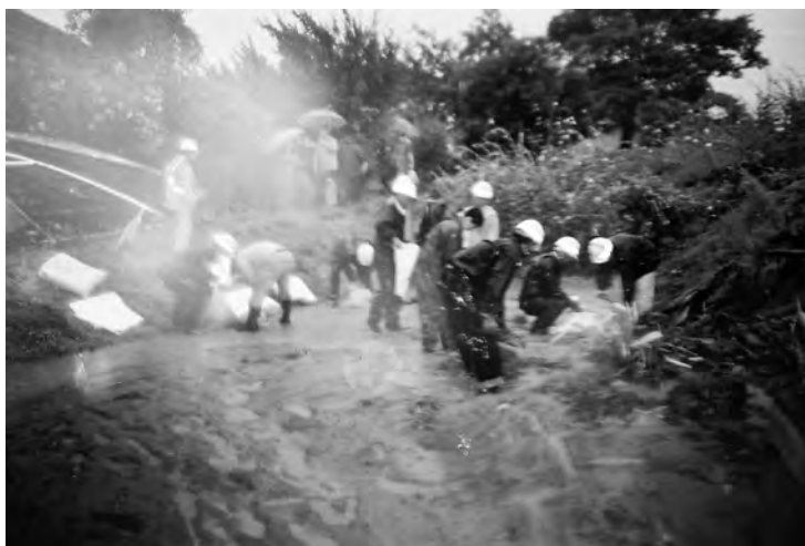
Photo 1. Flood-fighting activities to prevent water leakage of the levee.
