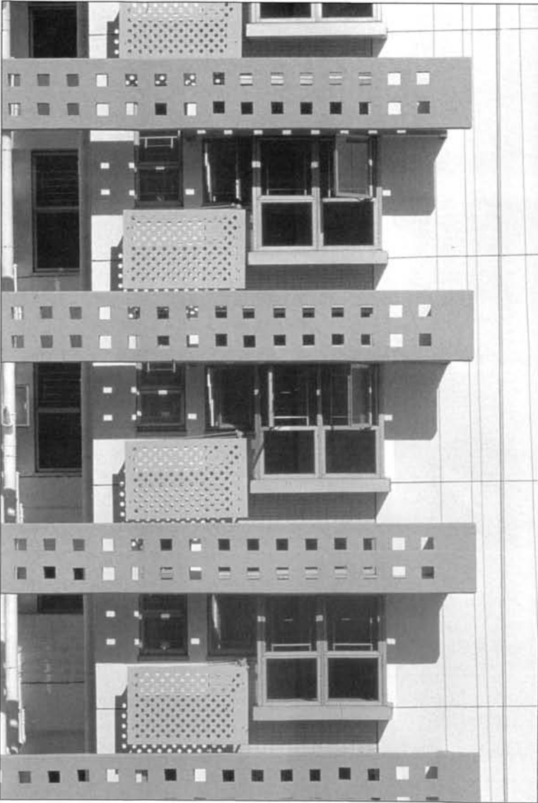
Plate 4 Elevation detail: External shading screen wall, bay window with upper light shelves, and perforated metal panel in front of clothes-drying racks.
