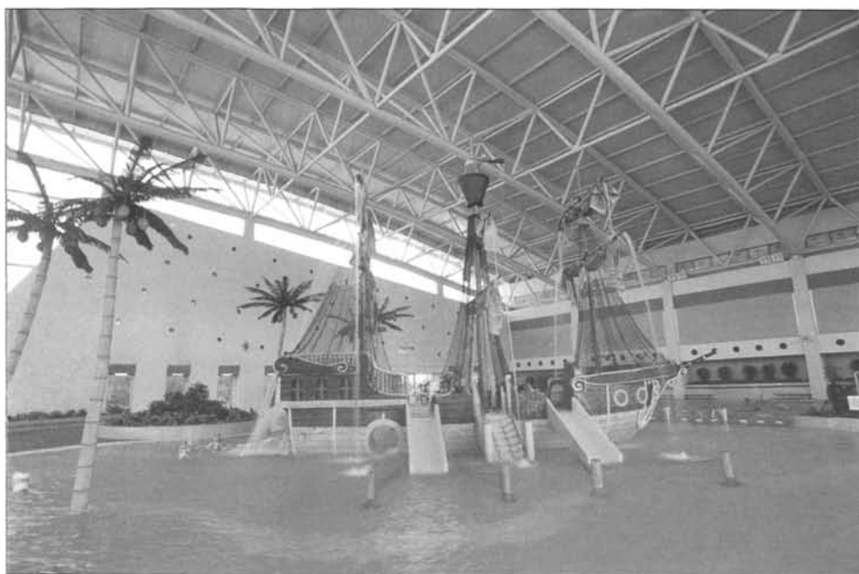
Interior of Hammer Hill Pool
