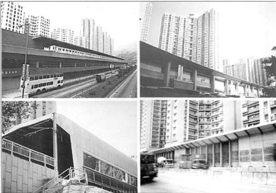
Plate 5 Noise barriers are among the most common mitigation measures adopted in Hong Kong.
