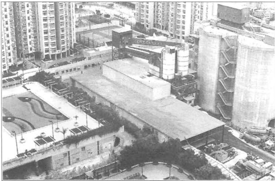
Plate 3 Proximity of flatted factories to residential buildings is aggravating the noise problem in Hong Kong (source: Environment Hong Kong 1998 ).
