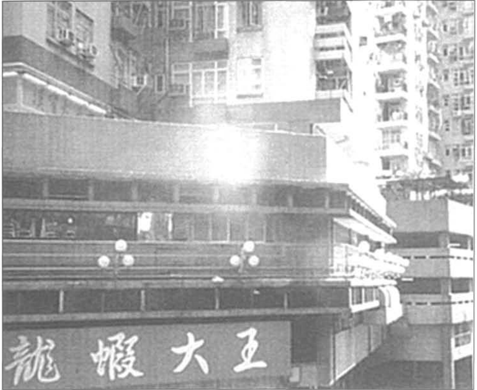
Plate 4 The problem of noise in a mixed-use environment in Hong Kong — a case of multiple dwellings sitting on top of a commercial podium (source: Environment Hong Kong 1998 ).
