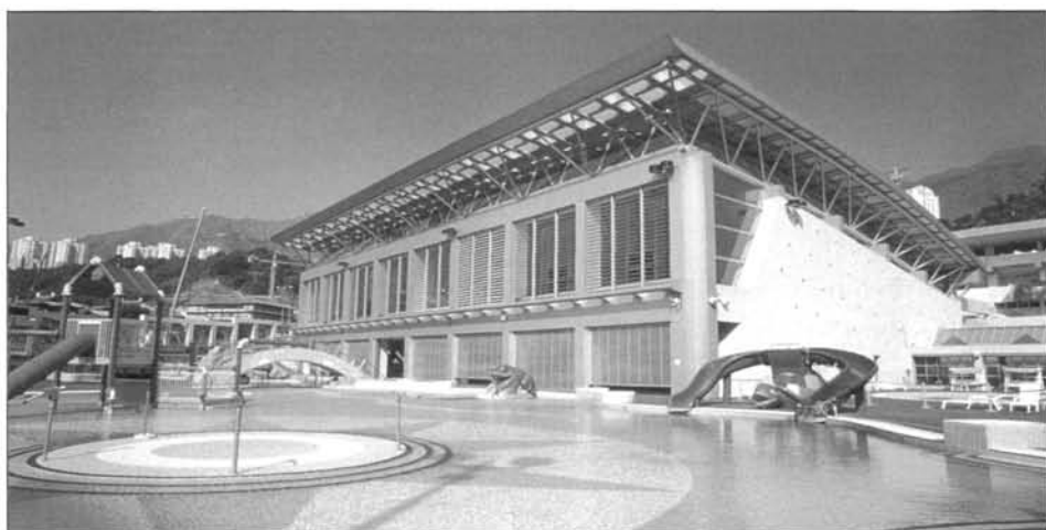
Exterior of Hammer Hill Pool
