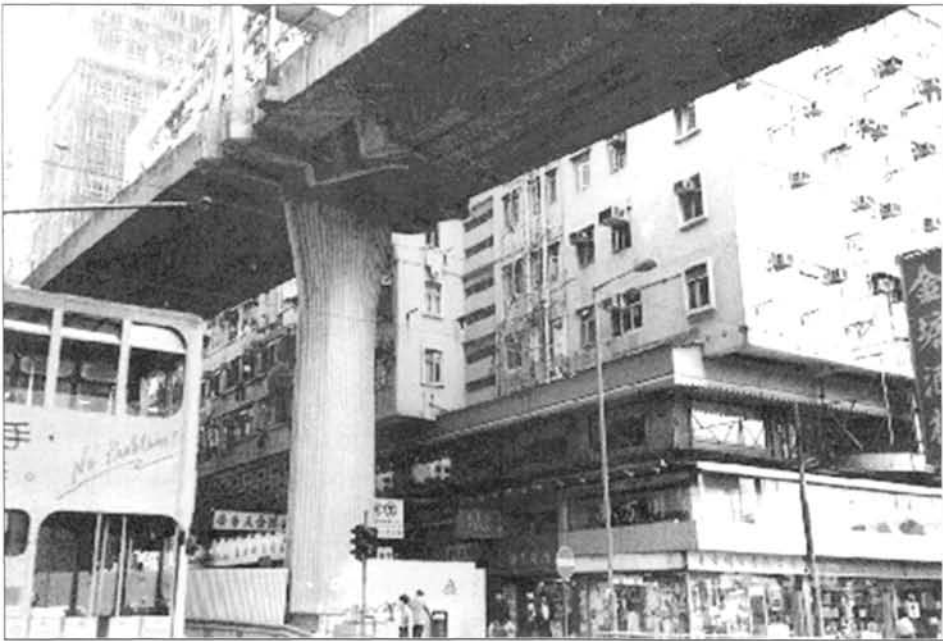
Plate 1 Lack of planning resulted in elevated roadways next to residential buildings.
