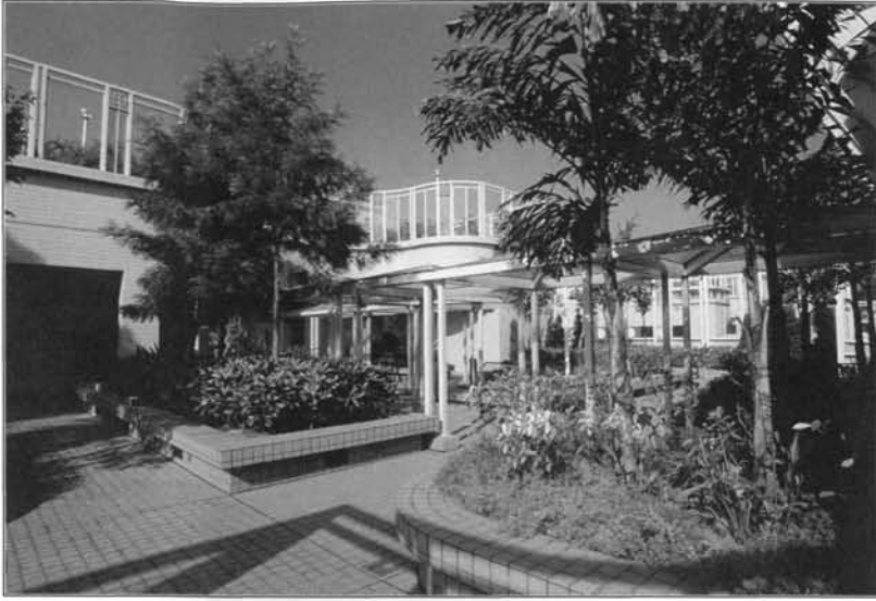
Roof Garden to Assist Thermal Insulation
