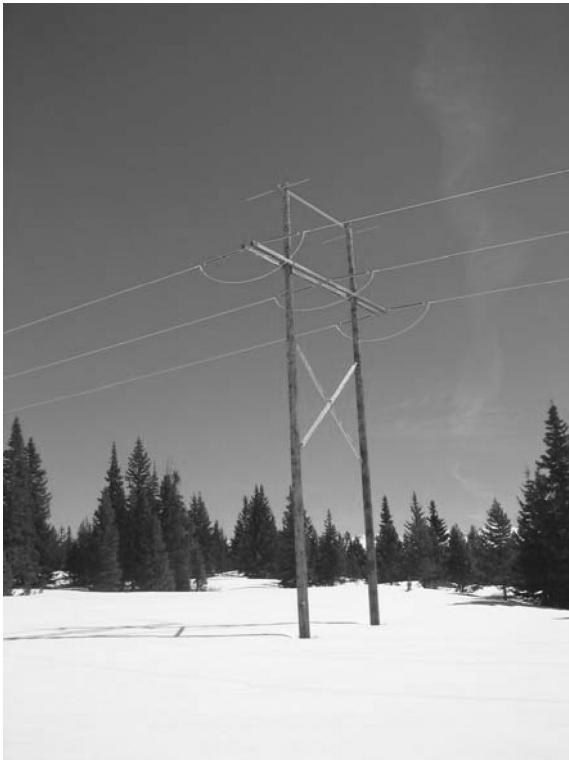
FIGURE 19.1 220 kV line with H-frame wooden towers.
