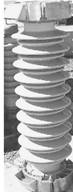
FIGURE 10.8 Post insulators.
