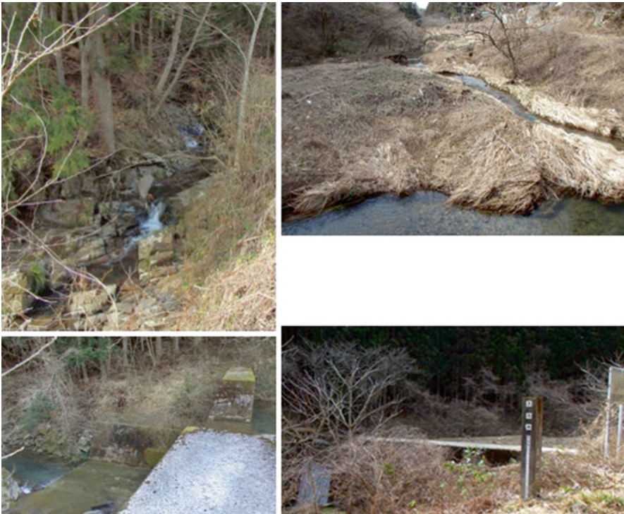
Fig. 12.4 Early Minatogawa River uppershed sediment control dam
