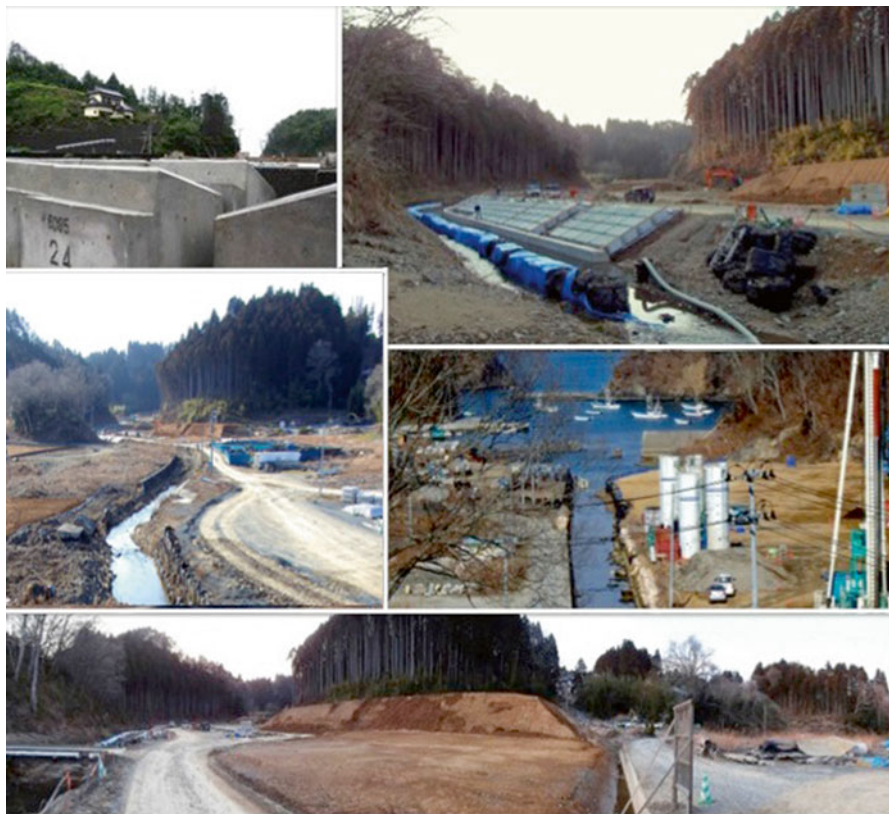
Fig. 12.16 Levee construction as of March 2015. Wide roads, concrete slabs, construction and drilling equipment as well as soil mounds are common sightings along the Minatogawa River shores
