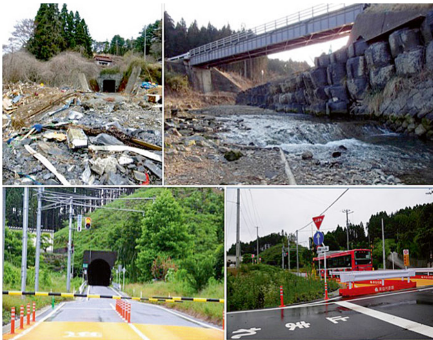
Fig. 12.15 Remains of the former JR Sanriku railways line and the new JR bus line crossing over the Minatogawa River
