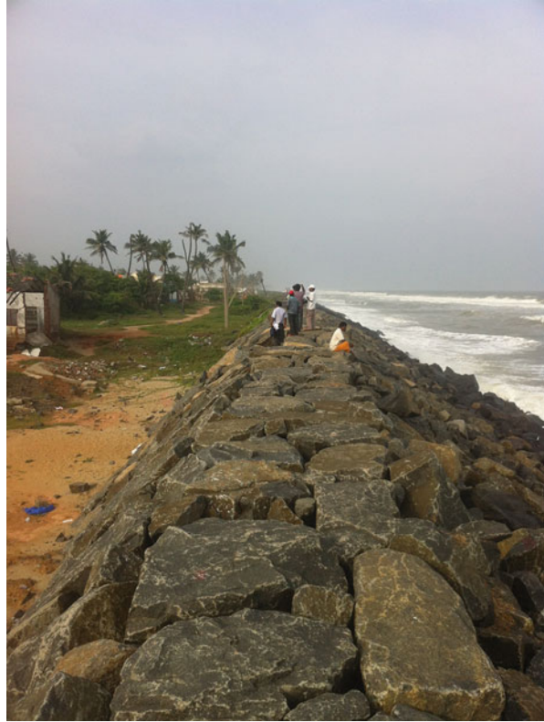
Fig. 7.7 Photo of the beach at Thevanampattinam (December 2013) is now occupied by a rubble mound sea wall. The approximate location of the sea wall is marked on the profile (Note that no beach is visible along the sea wall even at low tide)
