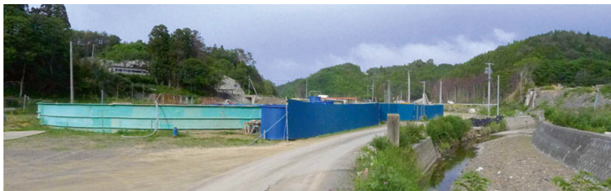
Fig. 12.13 Silver salmon fry aquaculture facility built on the Minatogawa riverside. A large accumulation of tsunami mud and debris on the exposed riverbed can be spotted
