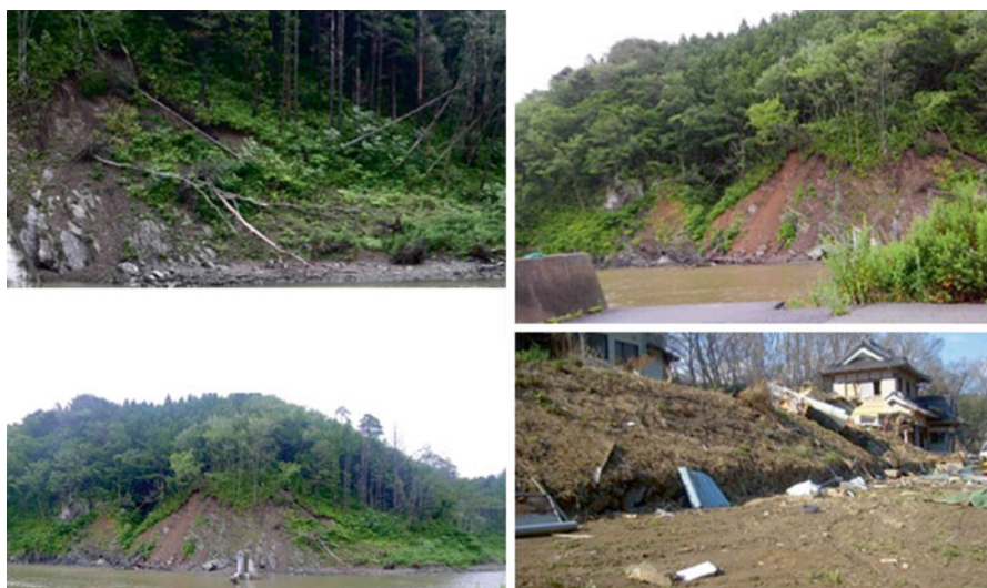
Fig. 12.9 Landslides and ground sinking along the Minatogawa River lowershed
