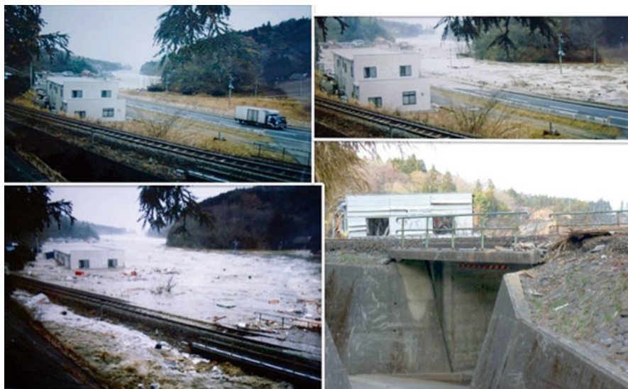
Fig. 12.5 First tsunami wave flowing through the Minatogawa River reaching Route 45 (photos provided by a local citizen), and the 3 m fully submerged underpass
