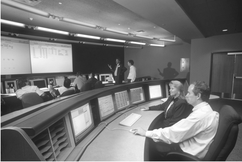
FIGURE 17.1 Manitoba Hydro Control Center in Winnipeg, Manitoba, Canada. (Photo used with permission of ALSTOM ESCA Corporation.)
