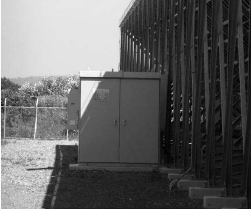
Figure 8.39 Actual box of a power conditioning system [30]
