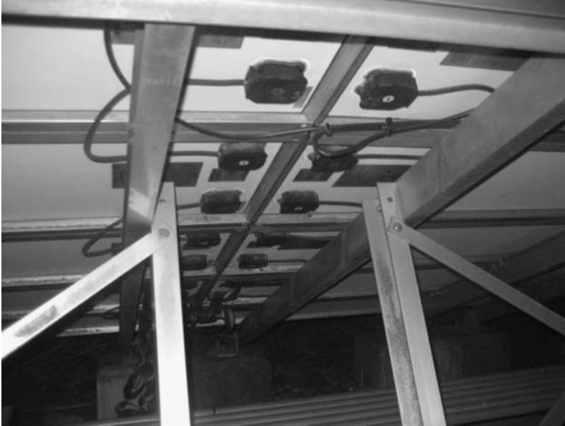
Figure 8.65 PV module wirings [37]
