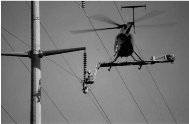
FIGURE 2.15 A lineman working from a helicopter platform.
