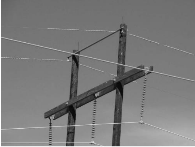
FIGURE 2.24 A pole-top view. (Courtesy of West Power Inc.)
