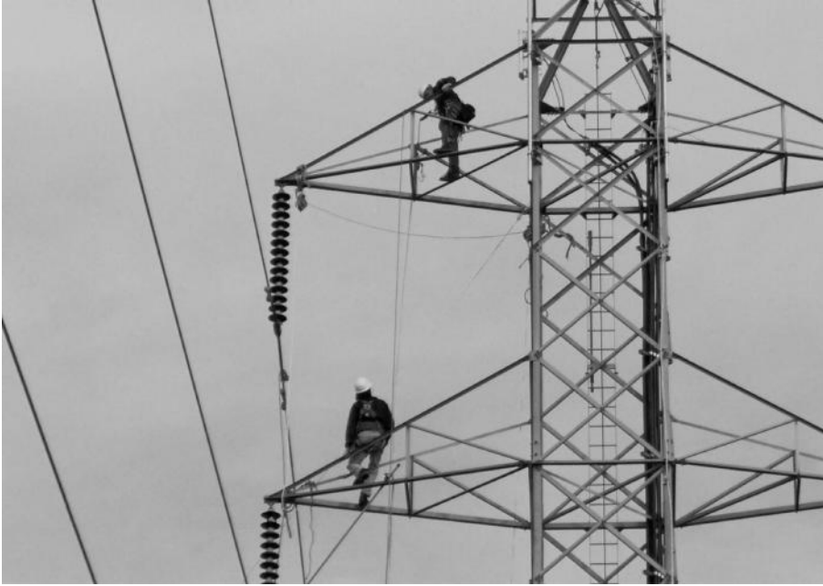
FIGURE 1.4 A transmission line is being upgraded.
