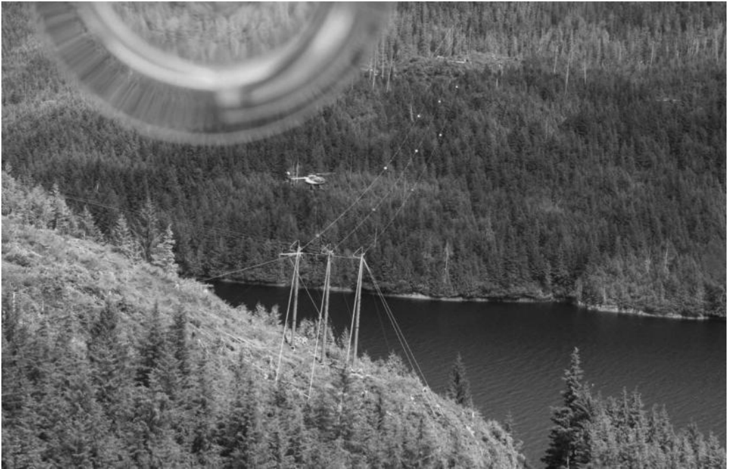
FIGURE 13.19 A river crossing of an HV transmission line.
