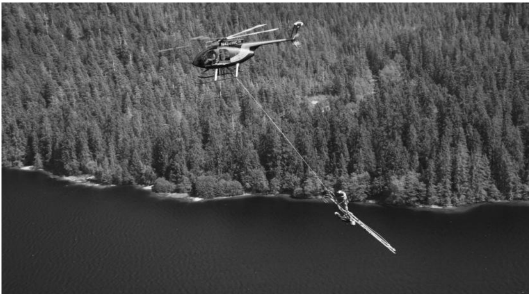
FIGURE 13.20 A helicopter carrying an incomplete pole to its location across a river.
