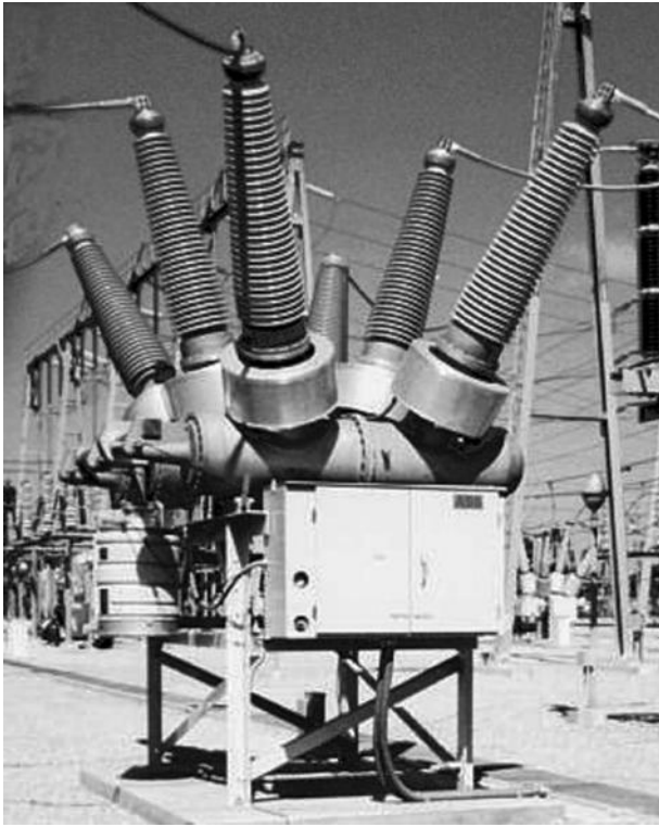
FIGURE 10.2 Three-pole-operated 245 kV SF 6 dead tank CB fitted with 80 kA interrupters. (Courtesy of ABB Corporation, Munich, Germany.)
