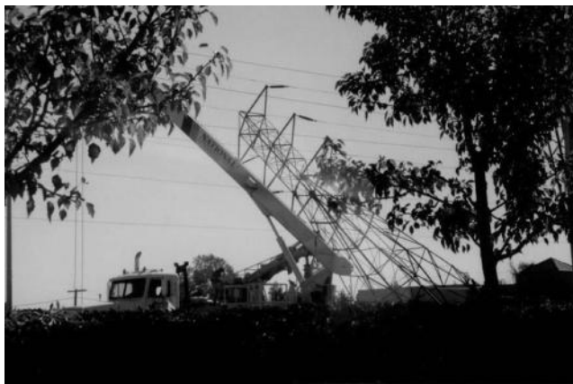
FIGURE 1.3 Installation of a 345 kV double-circuit transmission tower made of steel cage.
