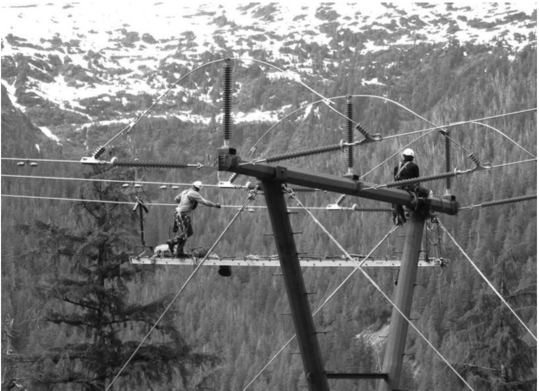
FIGURE 13.22 A crew is working on pole-top construction.
