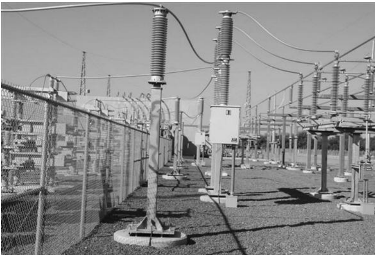
FIGURE 10.3 Single-pole-operated 138 kV SF 6 live tank CBs. (Courtesy of ABB Corporation, Munich, Germany.)
