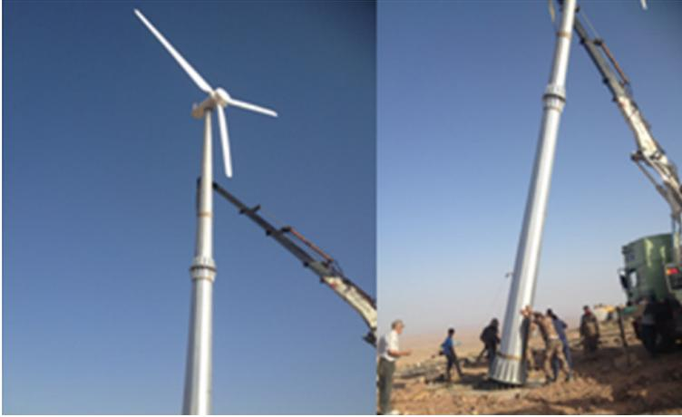
**Figure 7.12.** Free-standing tower for 20 kW wind turbine.
