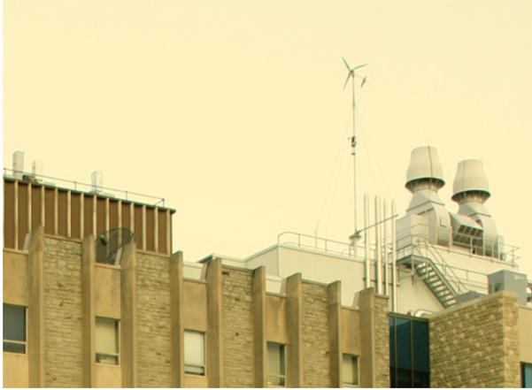
**Figure 5.4.** A small HAWT installed on the rooftop of the Western University Engineering building.
