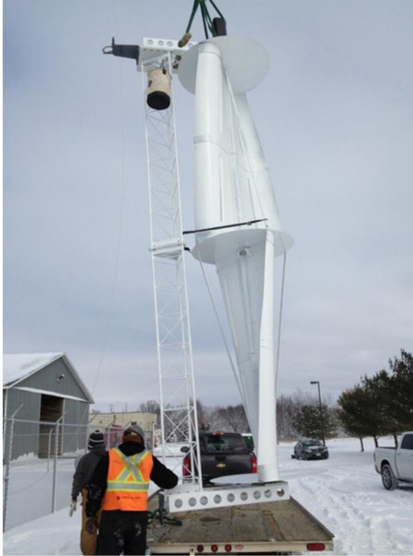
**Figure 2.5.** A small-scale wind turbine designed for telecommunication base transceiver stations during installation on a USA Department of Transportation telecommunication tower, 2012.
