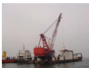
Fig. 1 320t pipe-laying crane
