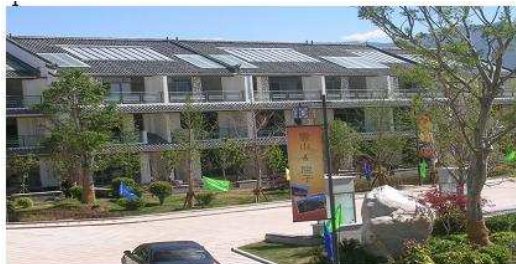
Figure 6 The sloping roof-mounted solar collector heat instance
