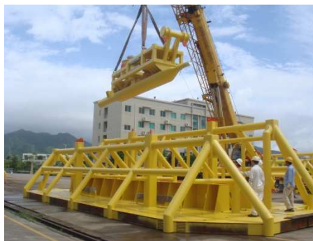
Fig.5. As-built PLET
