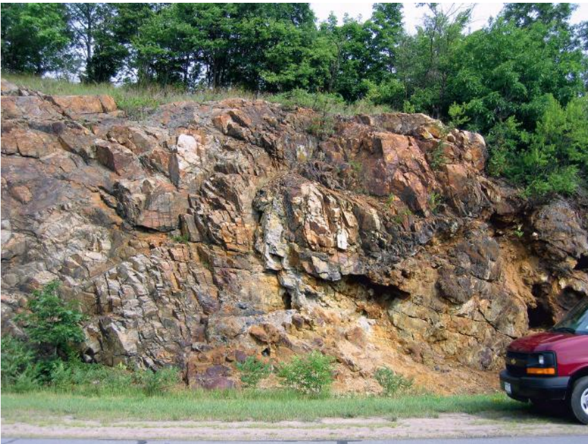
Figure 19.5 Hydrothermally altered and mineralized fracture zone in quartzite. More or less fresh quartzite is to the left, and the alteration zone is to the right, with rusty staining from the weathering of sulfides. The deep pit just above the hood of the vehicle is where a mass of sulfide has weathered out. Wellesley Island, St. Lawrence River, New York, USA.
