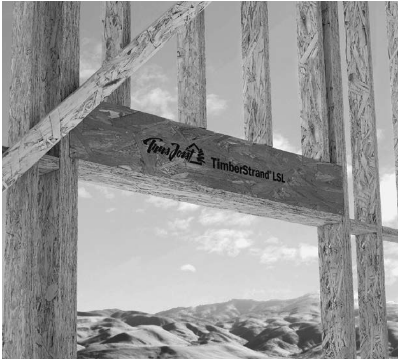
Figure 2.12 Laminated strand lumber (LSL) in header application
