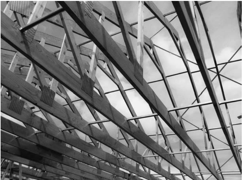
Figure 9.16 Truss plate (a) showing teeth, and (b) installed on a light framed truss Source: Image courtesy of Simpson Strong-Tie ©
