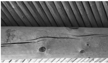
Figure 2.29 Common timber discontinuities: (a) knot, (b) split, (c) check, and (d) shake
