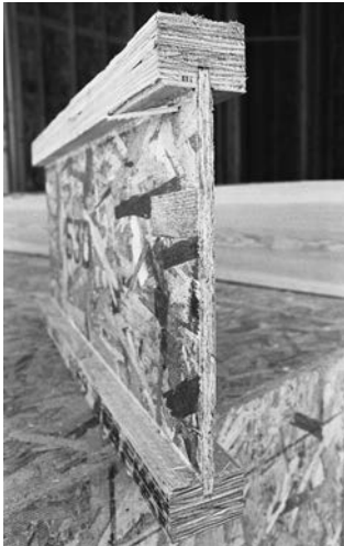
Figure 2.14 I-joist cross section with LVL flanges and OSB web
