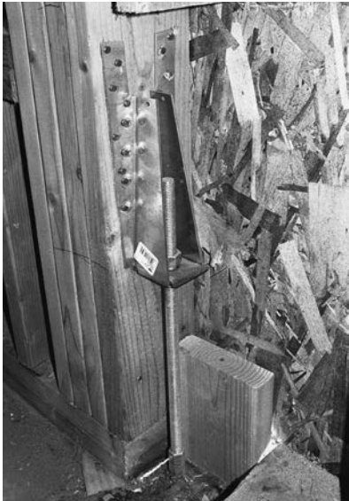
Figure 9.15 Shear wall hold down
