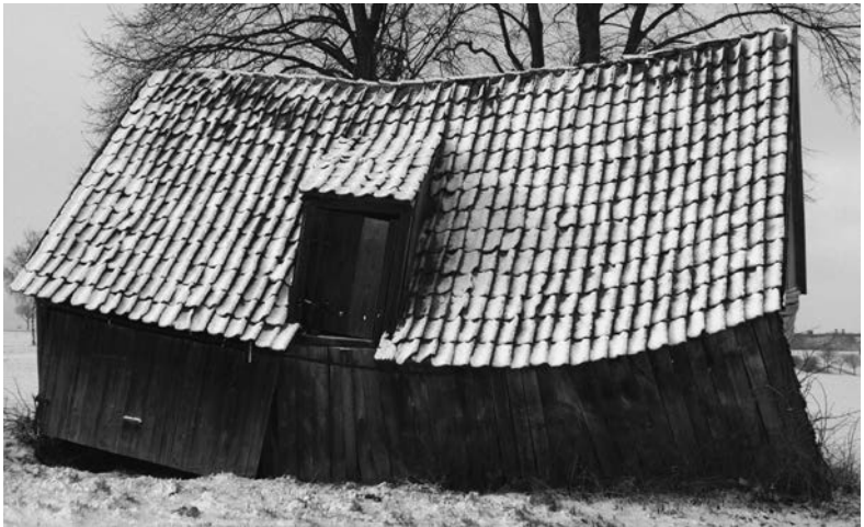
Figure 4.10 Old barn showing creep deformation
