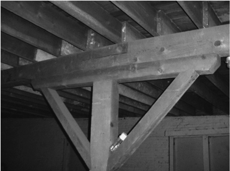
Figure 2.33 Post and beam in historic construction
