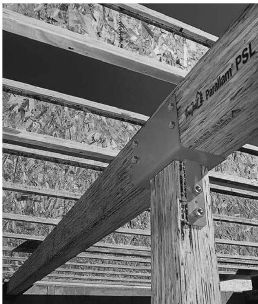
Figure 2.11 Parallel strand lumber (PSL) in beam and column application
