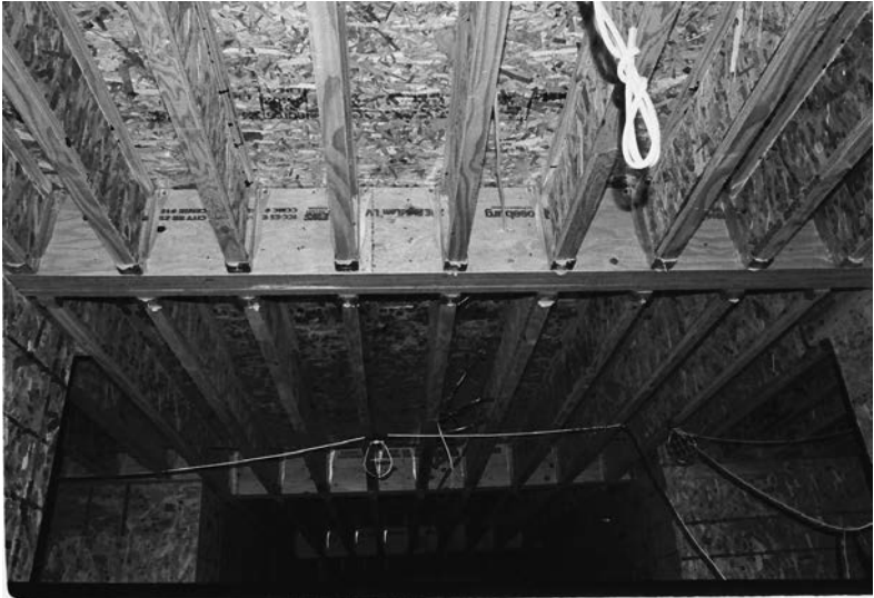
Figure 4.1 I-joists and LVL beam in new multi-family construction
