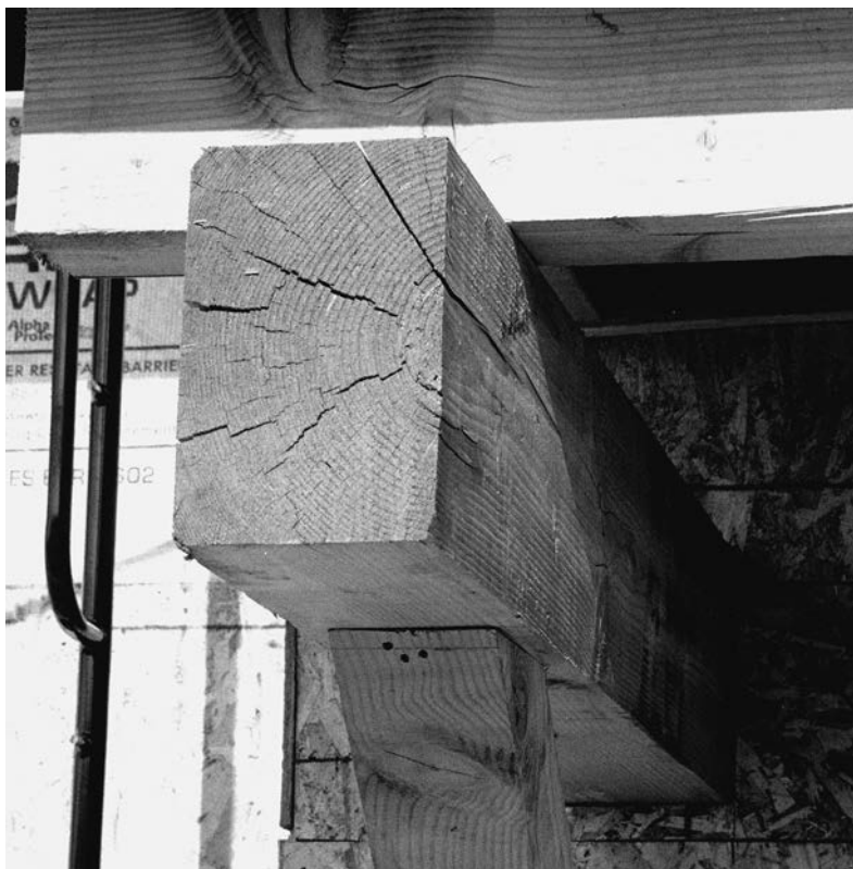
Figure 2.7 Dressed lumber in porch canopy
