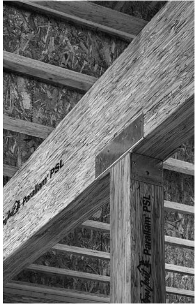
Figure 6.2 Structural composite lumber (PSL) column
