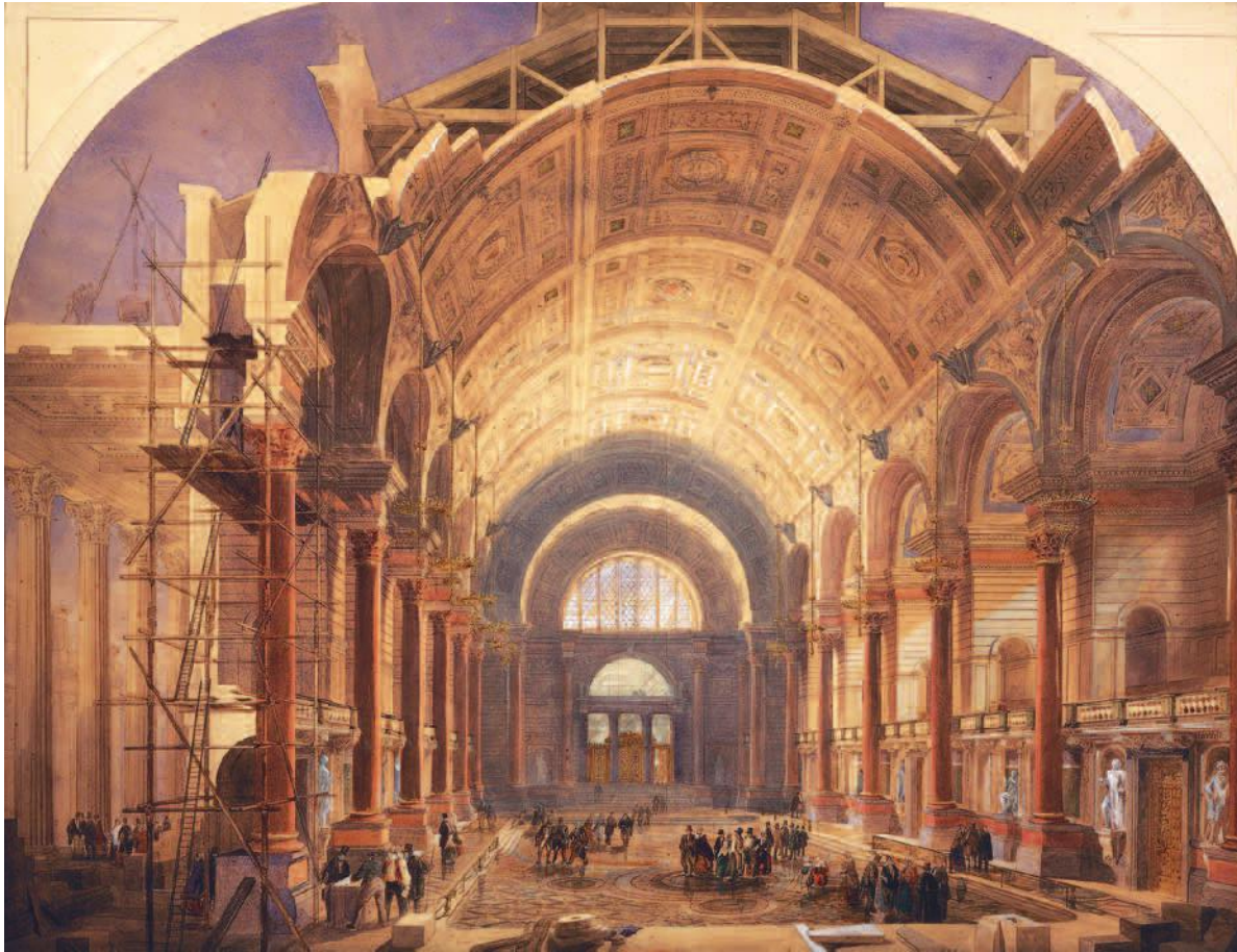
3 C.R. Cockerell (drawn by G.E. Goodchild, c.1854), Fantasy of St George's Hall, Liverpool, under Construction , Published with the permission of the National Museums Liverpool
