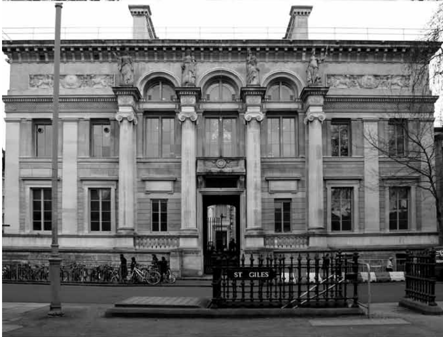
5.6 Comparison of a courtyard and street elevation at the Ashmolean Museum and Taylorian Institute, Oxford (photographs by Sonya Jensen, with permission from the Ashmolean)
