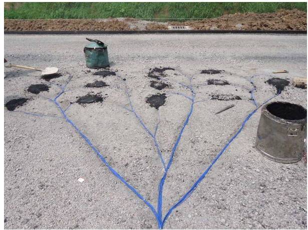
(b) Full view of installation
