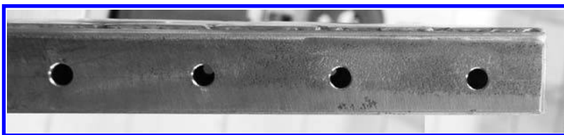
Fig. 10.23 Evacuation holes drilled in the end stops of the restraining-plate.
