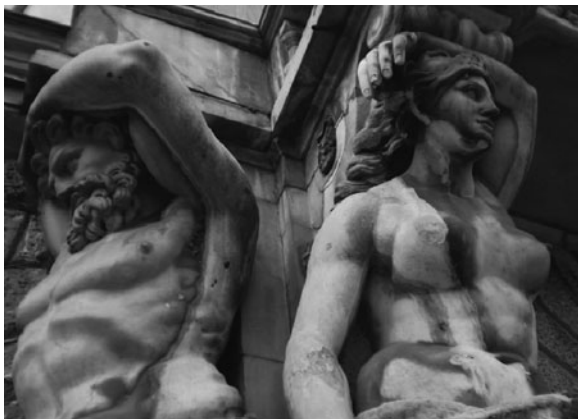
Fig. 1 Gypsum-rich patina on Manufacturer Demidov house in Saint Petersburg, arch. O. Monferan
