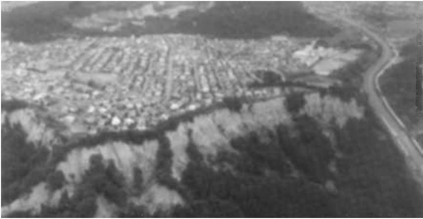
Fig. 7.1. Landslides of unwelded pyroclastic flow, Shirasu, Kyushu, Japan. (Photo by Kokusai Koku Photo.)
