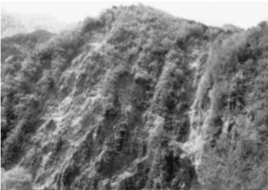
Fig. 7.12. Rockfall at the Toyohama Tunnel, Hokkaido, Japan. Dark areas on the detachment scar are wet areas.
