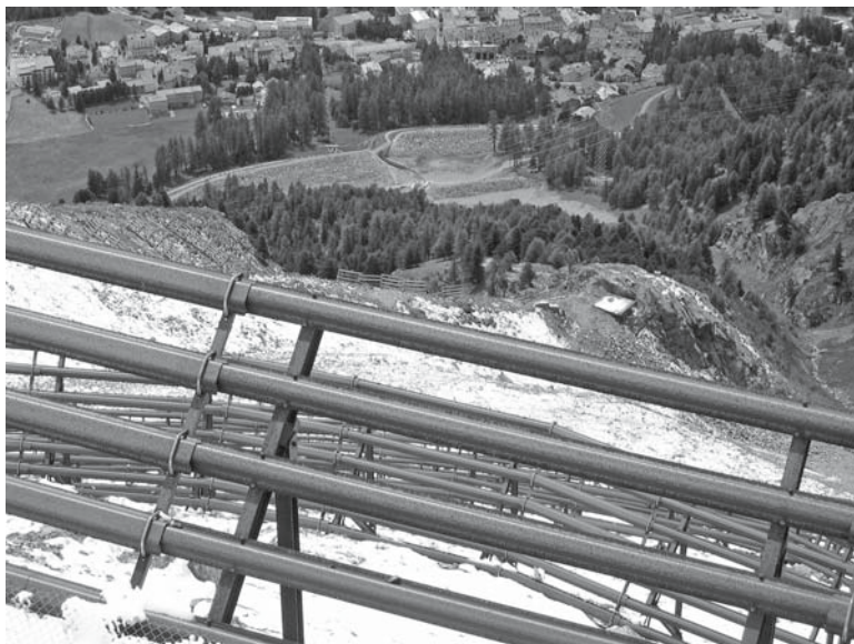
Fig. 14.10 Avalanche protection above Pontresina, Grisons Alps, Switzerland. The retention dam at the bottom of the slope is to protect against snow avalanches and debris flows from marginal permafrost (photo: W. Haeberli 2007)
