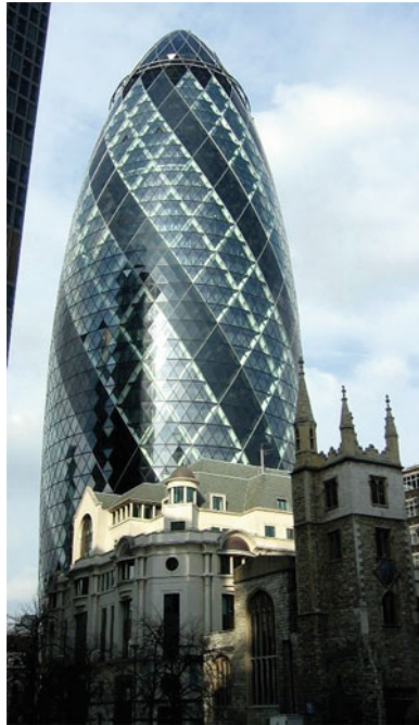
Norman Foster building, 30 St. Mary Axe (Photograph from Foster & Blaser (1993) – reproduced with kind permission from Springer Science + Business Media B.V.)
