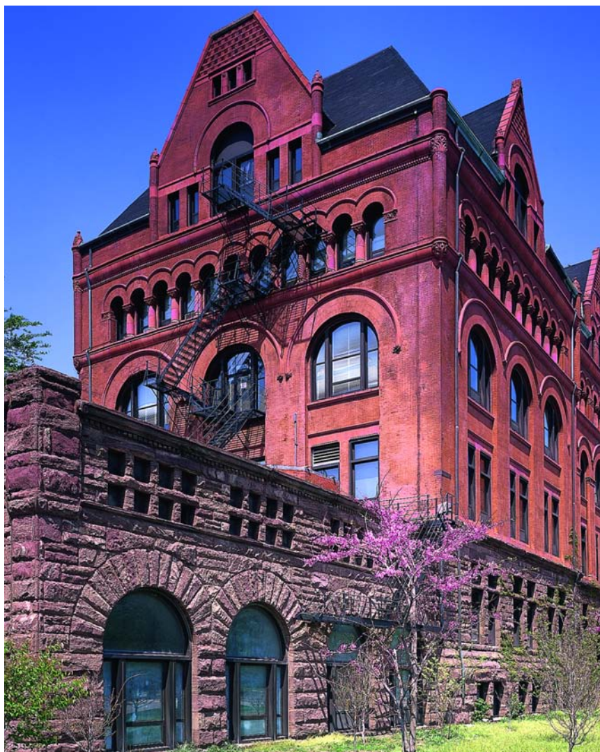
Original IIT Boiler Plant
