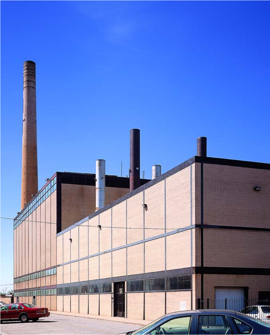
IIT Cogeneration Facility (right) with Boiler Plant (left)
