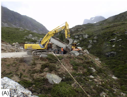
FIGURE 8.49 (A) Advanced filling construction with direct-shifted sods integrating structural elements such as boulders and dwarf shrubs. The sods and their root horizons are removed from behind the excavator as the filling gains height. (B) Sod mosaic with irregular gaps 1 year after direct-shifting. Before the emergence of complete vegetation cover through the expansion of the autochthonous flora, small-scale erosion and accumulation of soil material within the gaps may occur. These processes can be accepted as they contribute to site-specific heterogeneity. Source: photos: N. v. Albertini.
