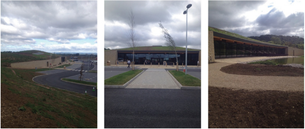
Figure 19.2 Views of the newly built Gloucestershire southbound MSA (M5).
