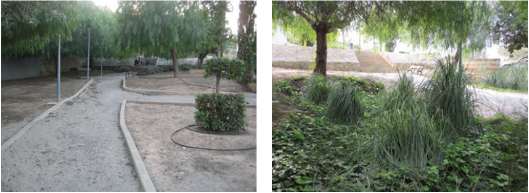
Figure 26.6 Costa Ermita park before (left) and after (right) retrofitting three infiltration basins.
