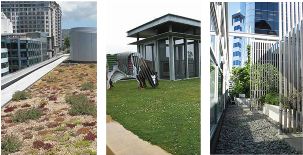
Figure 28.3 Green roofs are relatively uncommon in New Zealand. The New Zealand green roofs shown increase in depth and cost from left to right: Auckland commercial building with lightweight sedum and succulent roof; Auckland café turf roof with sculpture and lift; Wellington commercial building roof garden.
