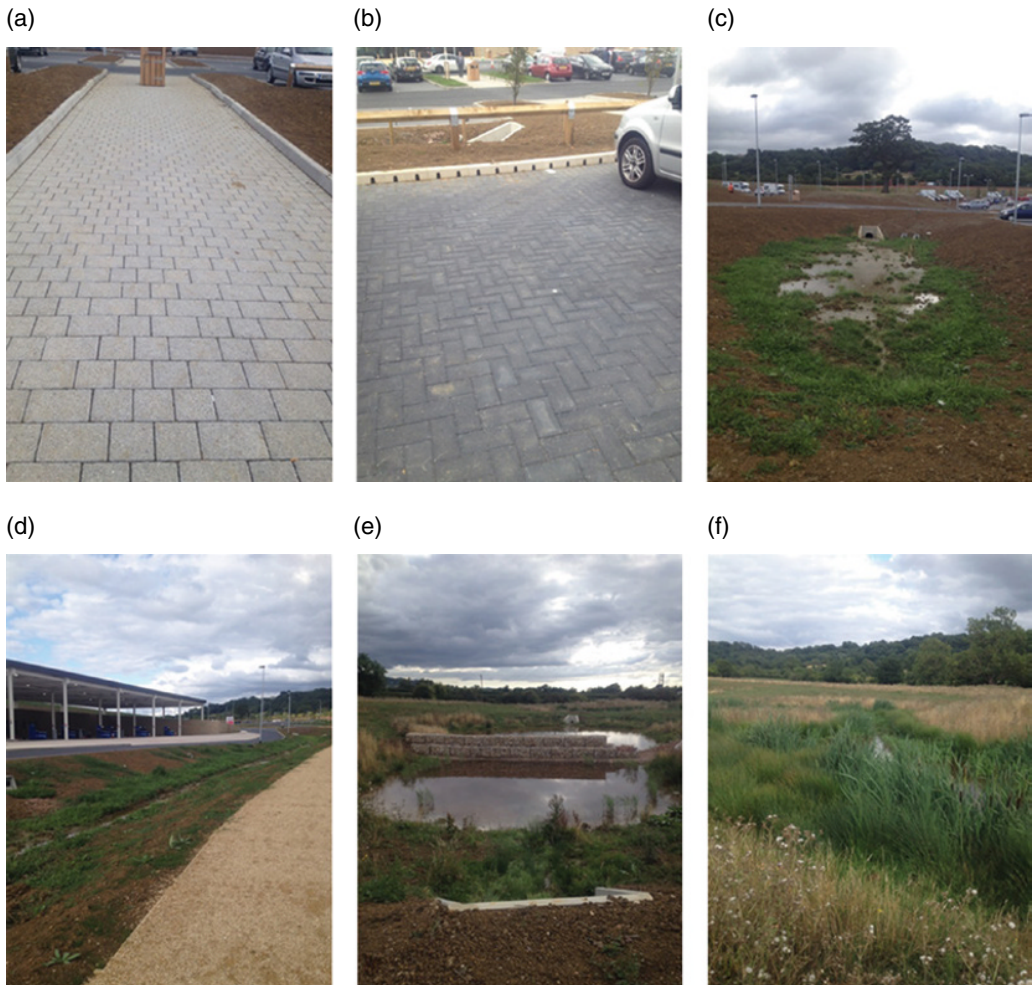
Figure 19.3 Devices used for the SuDS management train at the newly built Gloucestershire southbound MSA (M5).
