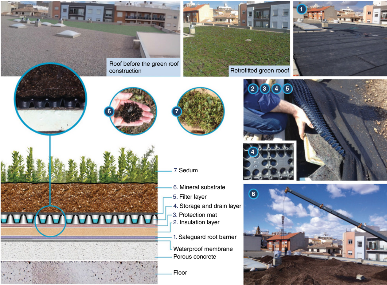
Figure 26.9 Retrofitting a green roof in Benaguasil: construction stages and roof layers.
