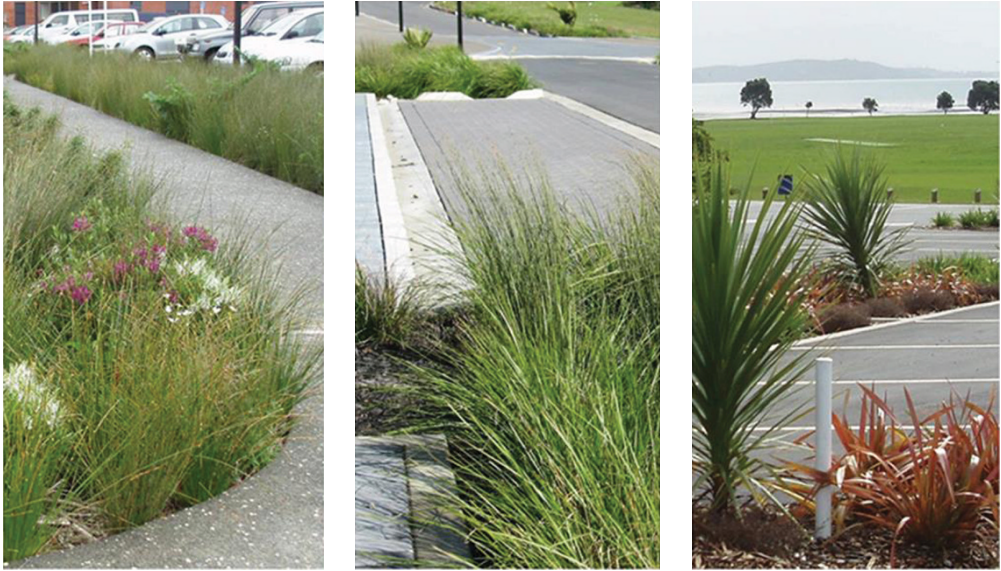
Figure 28.1 Densely planted rain gardens and swales are the most common devices used in Auckland projects with WSD. Native plants are usually used in public spaces to reinforce sense of place.
