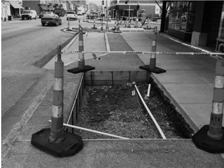
Figure 25.4 Retrofit construction in South Grand Boulevard, St Louis, Missouri.
