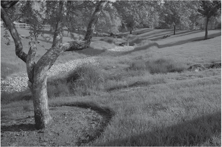
Figure 25.3 Infiltration basin in a suburban residential neighbourhood near Boise, Idaho.
