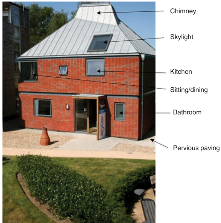
Figure 13.2 The EcoHouse, showing the location of the pervious paving.
