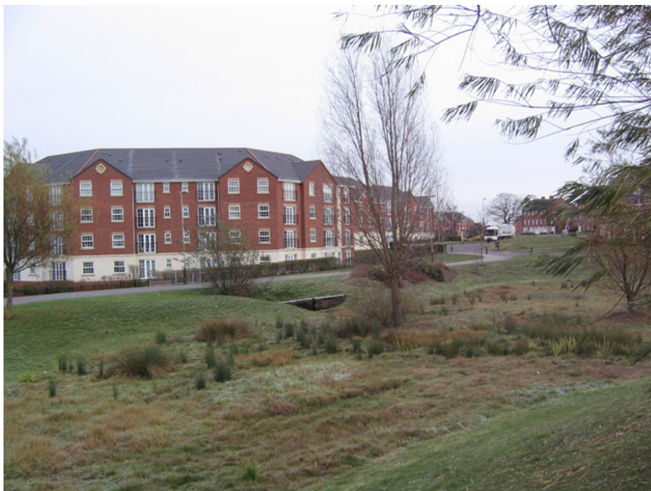
Figure 7.1 Wetland and swale in a housing estate, N. Hamilton Leicestershire, UK.
