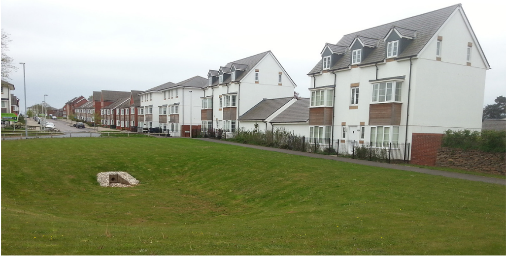
Figure 15.2 A typical SuDS solution used in England and Wales – a detention basin at Newcourt, Exeter, Devon, England.
