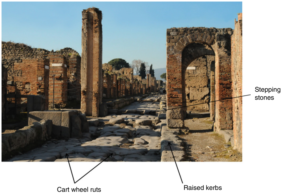
Figure 2.15 Pompeii raised kerbs with stepping stones.
