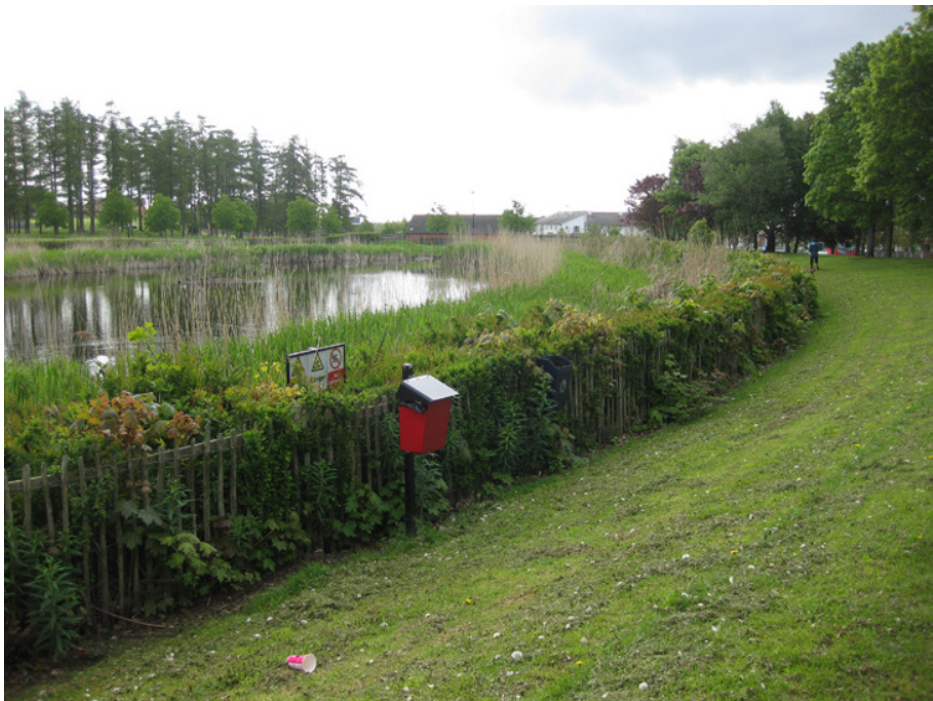
Figure 29.1 Fencing and fringing vegetation preventing access to open water around a SuDS pond, Scotland.
