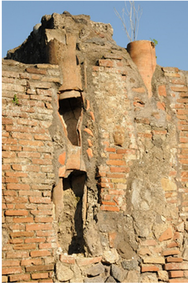
Figure 2.3 Terracotta pipe for rainwater harvesting from roofs at Pompeii, Italy. The pipes would have directed water into cisterns to service individual buildings.
