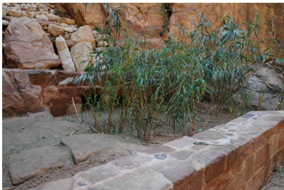
Figure 2.5 Stilling basin at the outlet of Wadi Jilf (Petra, Jordan). Bioretention is provided by the plants growing in the basin at the present day. Two outlets can be seen in the cross-drainage structure in the background.
