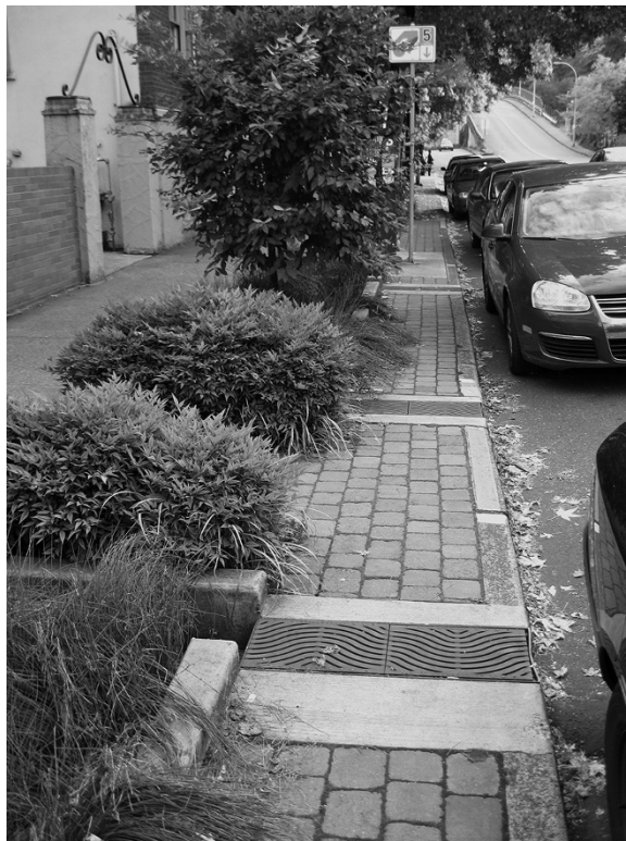
Figure 25.1 Rain gardens in Portland, Oregon.
