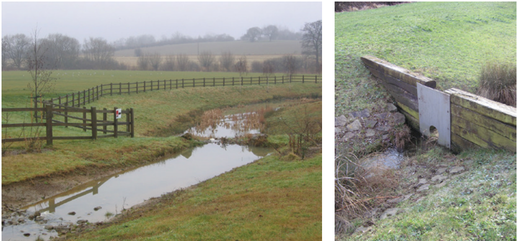
Figure 7.7 (left) Swale with leaky stone dam creating downstream wetland area, Oxfordshire, UK. (right) Wood and metal dam across a swale, N. Hamilton, Leicestershire.
