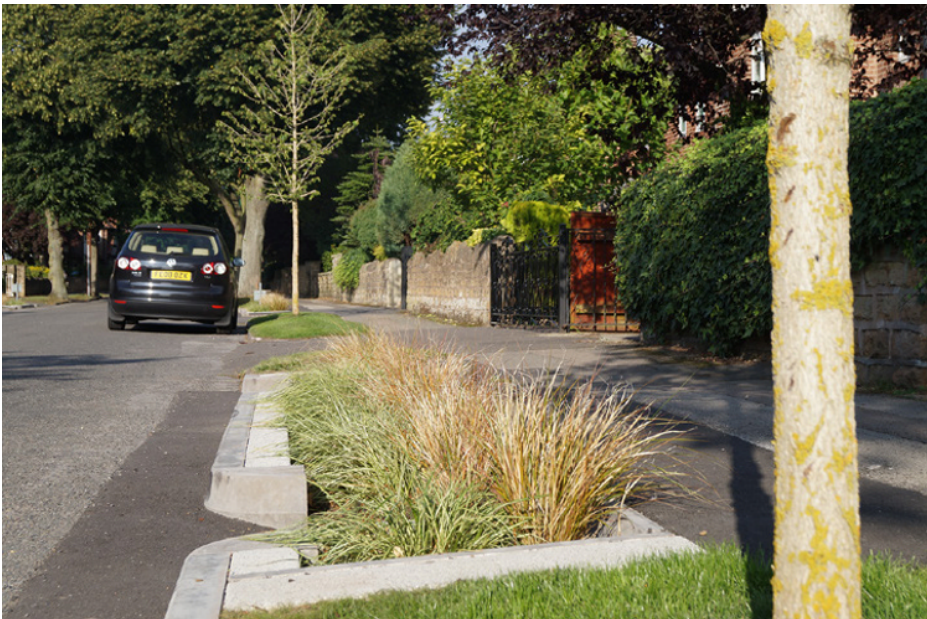
Figure 20.4 Daybrook rain garden, Nottingham, UK.
