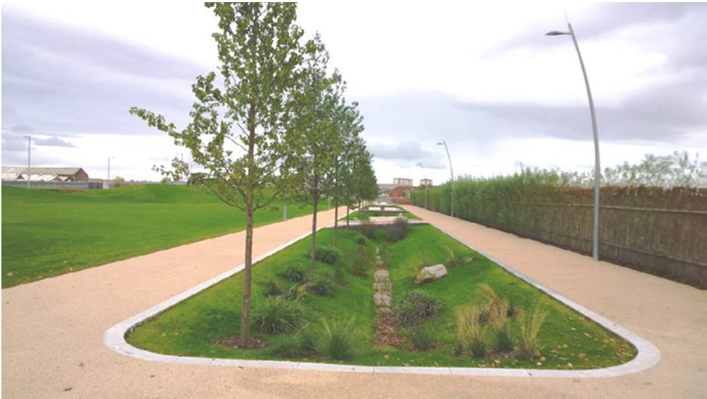
Figure 27.1 A new swale that will form part of a central amenity area in a new development Dalmarnock in the East End (courtesy MGSDP).
