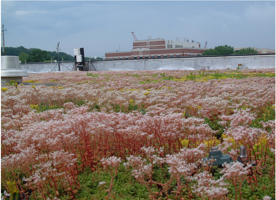
Figure 14.2 Extensive green roofs such as this one on the Plant and Soil Sciences Building at Michigan State University are generally built with substrate depths less than 15 cm. Because of the shallower depth, plant species are limited to grasses, herbaceous perennials, annuals and drought-tolerant succulents such as sedum. They have less potential to sequester carbon.
