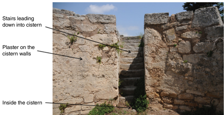
Figure 2.4 Cistern from Tylissos, Crete.
