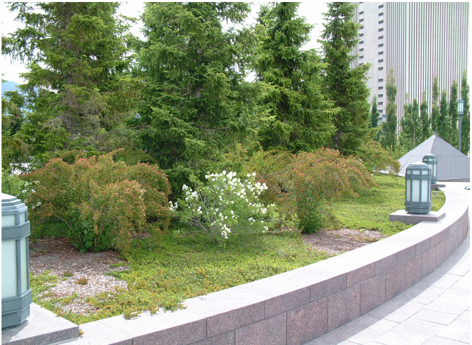
Figure 14.1 Intensive green roofs, such as the roof of the Church of Jesus Christ of Latter-day Saints Conference Center in Salt Lake City, Utah, include shrubs and trees, and appear similar to landscapes found at ground level.
