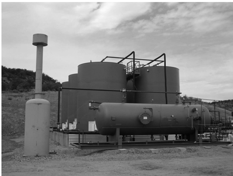
FIGURE 7.6 A typical oil field tank battery. (Photo courtesy of NIOSH and OSHA. Available from: http://blogs.cdc.gov/niosh-science-blog/2014/05/19/flowback/flowback2-4/ )
