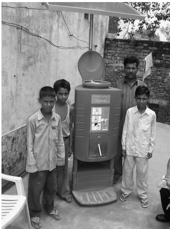
FIGURE 9.5 Naiade solar-powered UVC disinfection system on-site in India. (From Naiade 2015. http://www.nedap-naiade.com [accessed January 9, 2015].)
