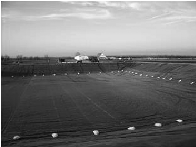
FIGURE 7.7 Freshwater pit with liners at the oil field. (Reprinted with permission from Unit Liner Co., Ltd. Fresh water pit with liners at the oil field . 2015; Available from: http://www.unitliner.com/frac_pit_liners.html .)
