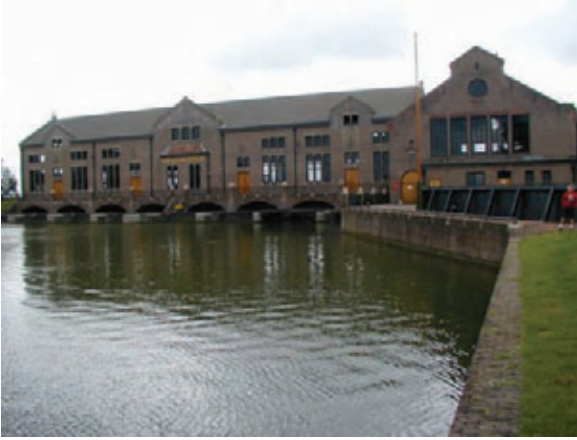
Figure 17.12. The Wouda pumping station was built to drain large areas in Friesland, Netherlands, and is the largest steam pumping station ever built. It is now on the World Heritage List.
