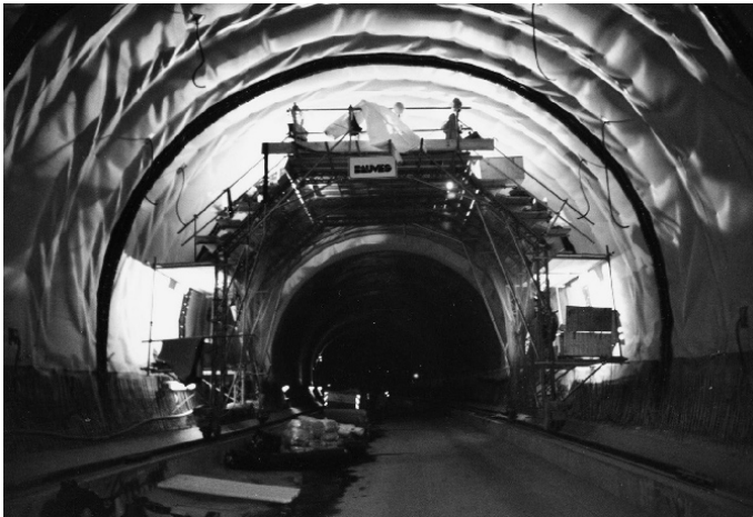
Figure 5-22 Plastic waterproofing membrane.
