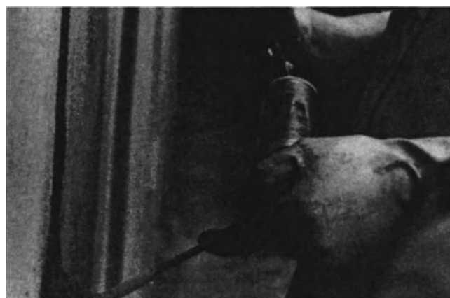
Fig. 27-25. Crack injection of chemical grout.
