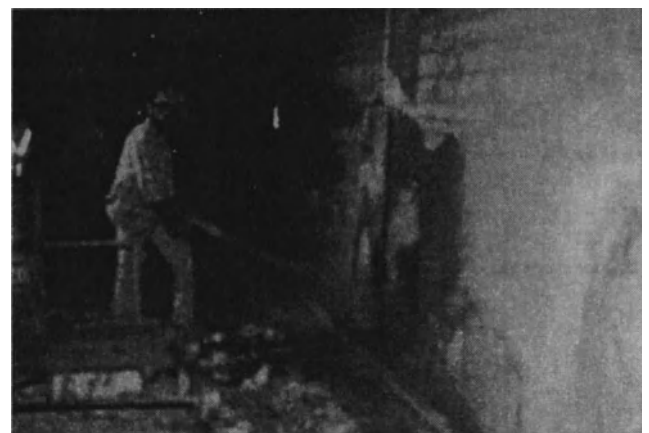
Fig. 27-19. Shotcrete application.
