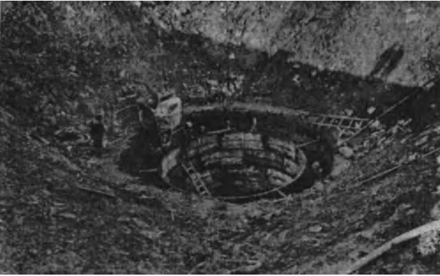
Fig. 10-5. Constructing shaft collar.
