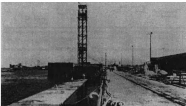
Fig. 14-21. Survey tower (Second Hampton Roads Tunnel).
