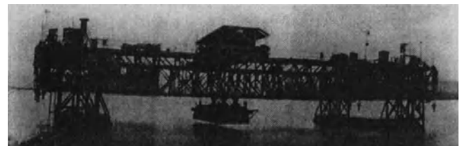
Fig. 14-20. Screeding rig—Trans-Bay Tube.
