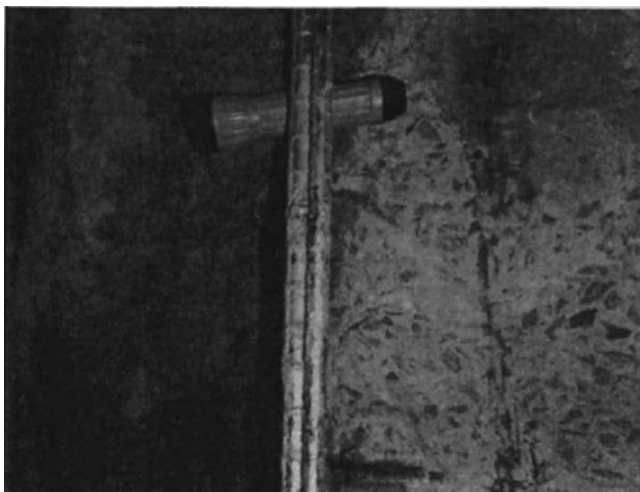
Fig. 27-16. Reinforcing steel (“white metal” condition).
