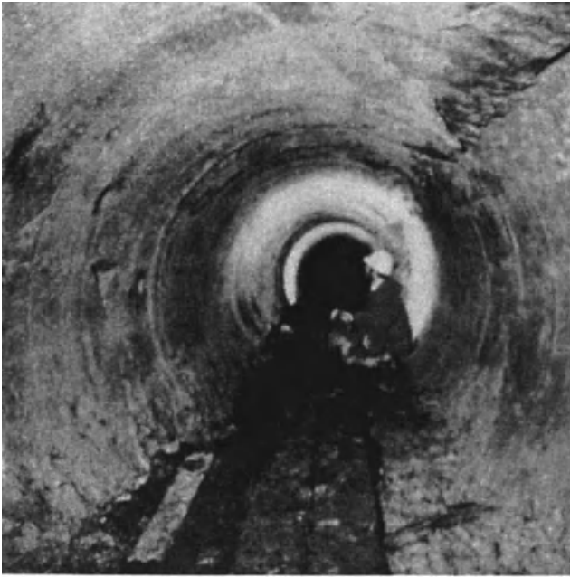
Fig. 11-2. Seven ft diameter trial tunnel driven in 1881 by Beaumont/English TBM at Abbotts Cliff. Unlined tunnel as it appears today.
