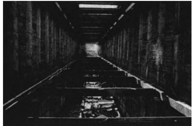
Fig. 17-10. Internally braced soldier pile and lagging walls, San Francisco Clean Water Program.
