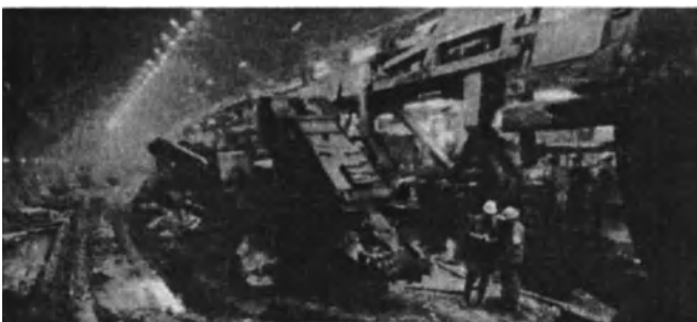
Fig. 11-9. Voest-Alpine AMT70 Roadheader after completion of Channel Tunnel UK crossover excavation. Robbins/Markham UK Running Tunnel TBM pauses in cavern before resuming drive toward France.
