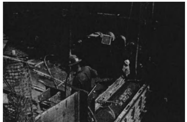
Fig. 16-6. A “stacked drift” lining.
