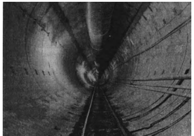
Fig. 5-11. Los Angeles Metro—segmented concrete construction lining.
