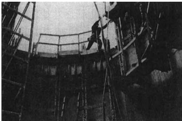
Fig. 9-16. Forms for concrete shaft lining.
