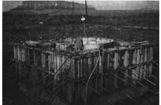
Fig. 10-6. External form walls.
