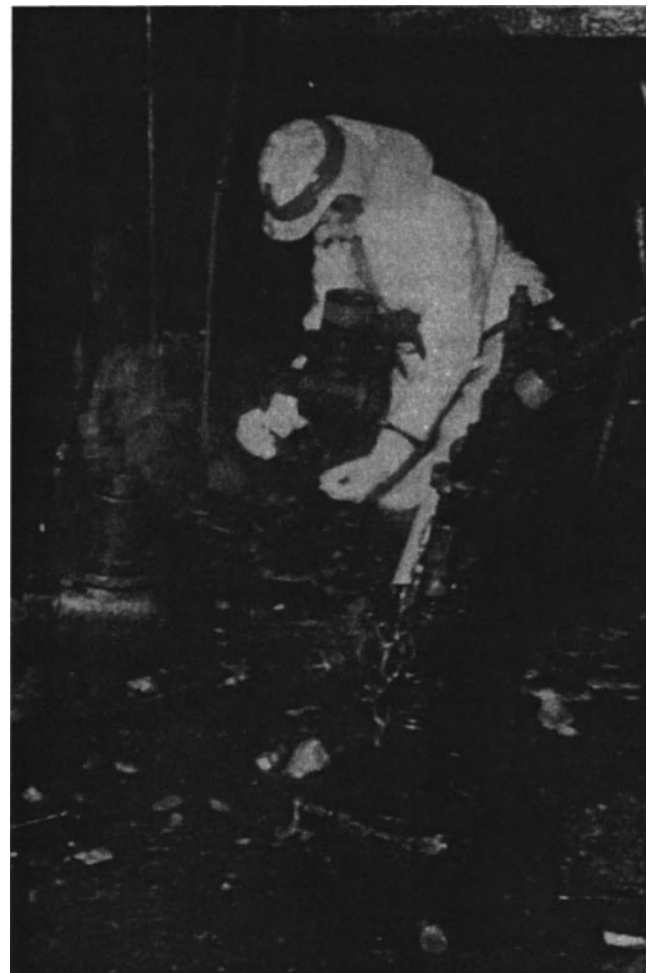
Fig. 10-14. Grout cover from the shaft floor against 1,300-psi hydrostatic head.
