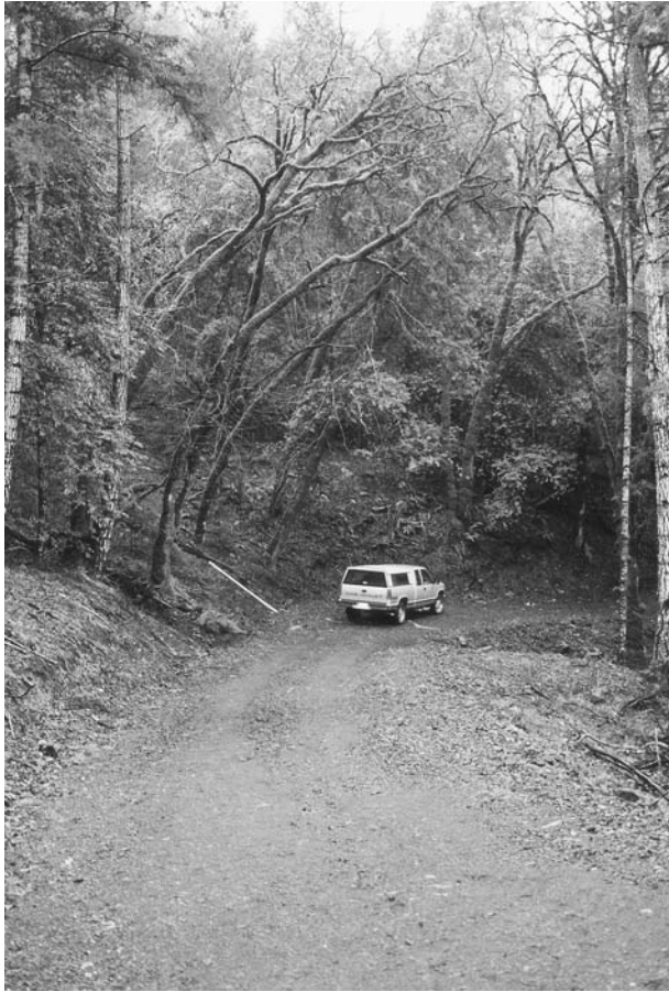
Photo 18 A well-designed permanent forest access road in Mendocino County, California, with a rocked surface. (Photograph by Walter Smith.)
