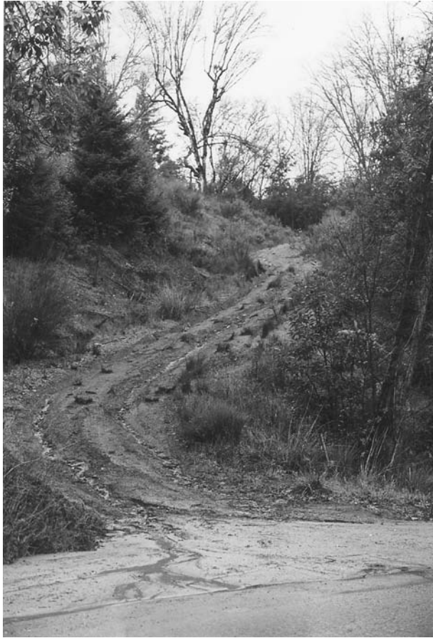
Photo 17 Although the state of California has the most stringent forestry practice laws in the U.S., people ignore the regulations and the state has poor oversight, as demonstrated by this logging road in Mendocino County without waterbars to control soil erosion. (Photograph by Walter Smith.)
