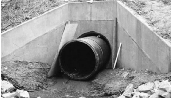
Figure 5-7. Inserted Pipe.
