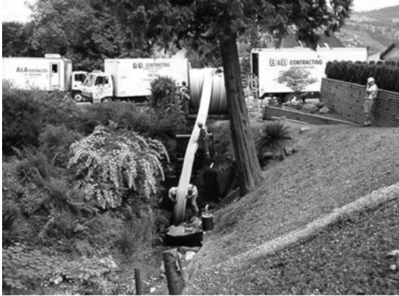
Figure 5-13. Lining a Culvert.
