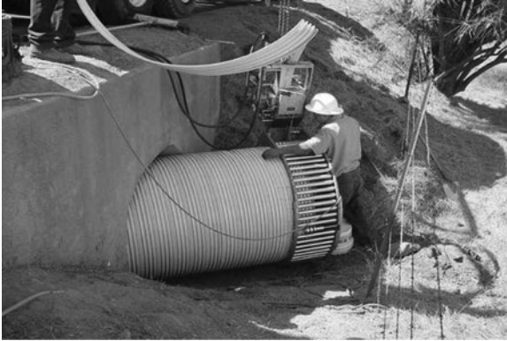
Figure 5-23. Spiral-Wound Stationary Winding Machine.
