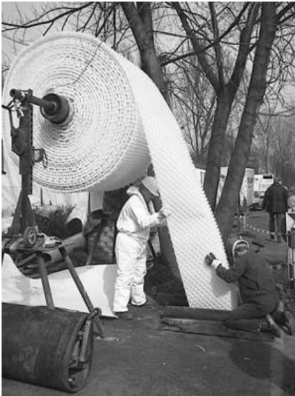
Figure 5-17. Insertion of the Anchored Liner.
