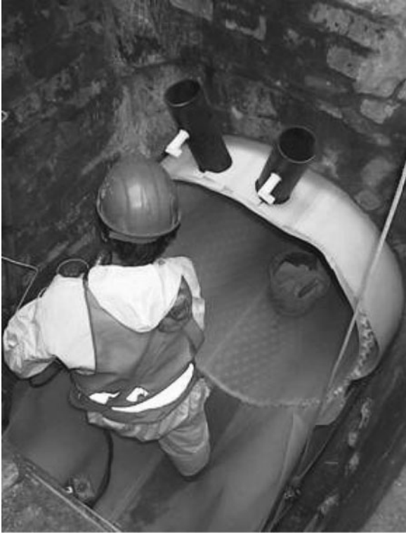
Figure 5-18. Attachment of Grouting Ports.
