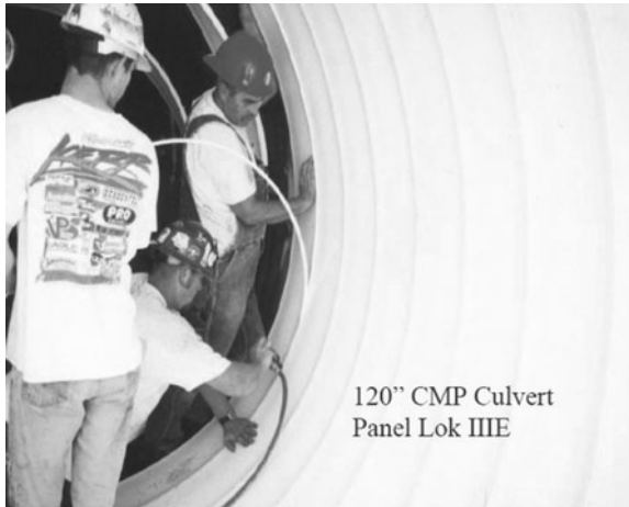
Figure 5-25. Manual Installation. Courtesy of Danby of North America.
