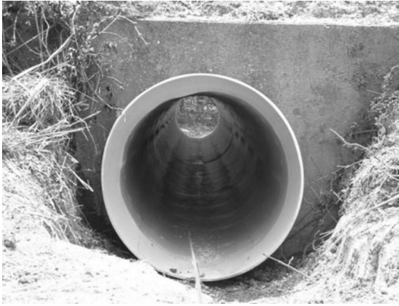
Figure 5-12. Culvert Renewed with a Thermoplastic Pipeliner.
