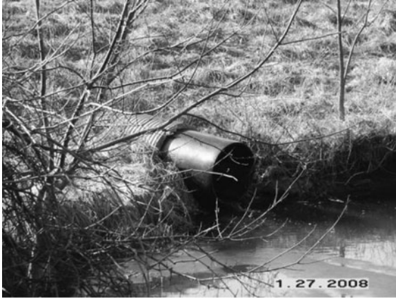
Figure 5-9. Sliplining Finished Product.
