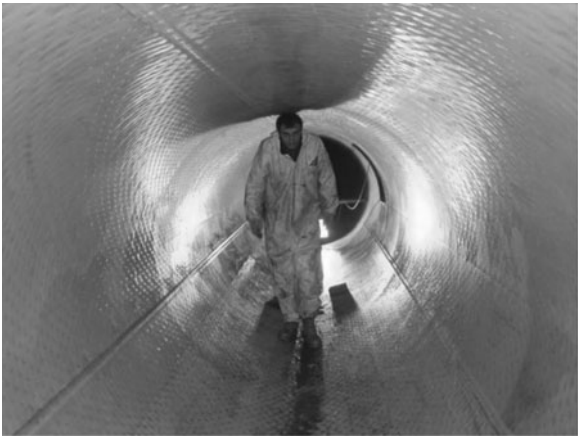
Figure 5-19. Completed HDPE GIPP Installation.
