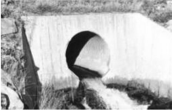
Figure 5-6. Metal Culvert with Paved Concrete Invert.
