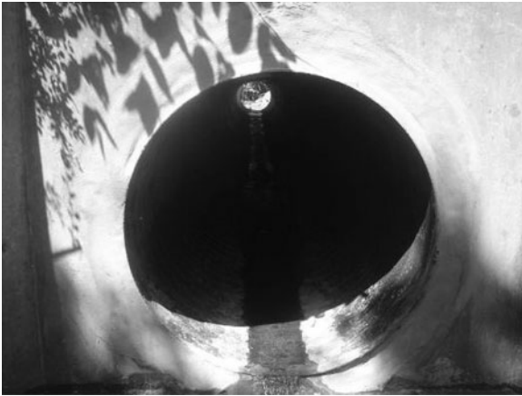
Figure 5-8. Grouted Pipe.
