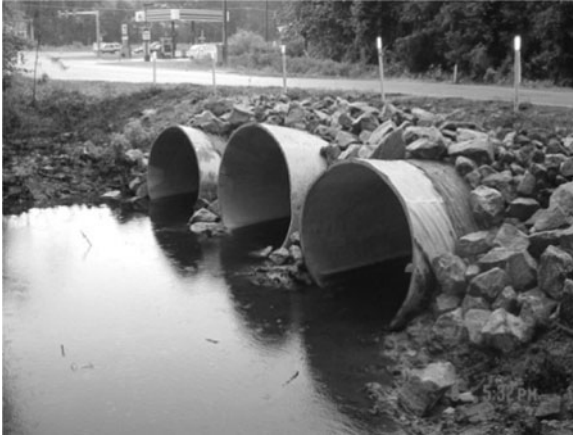
Figure 5-1. CIPP Finished Product.
