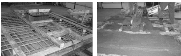
Figure 2 Fabrication of a test specimen
