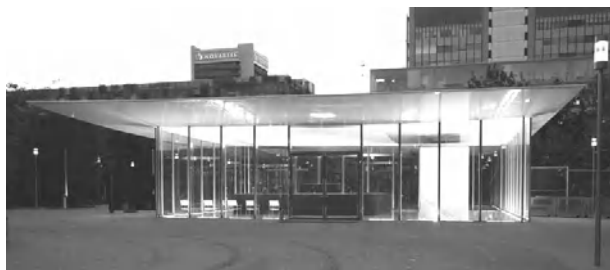
Figure 1 Novartis Campus Main Gate Building with GFRP cell-core sandwich roof (Keller et al. 2008)
