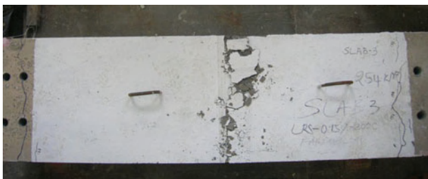
Figure 4 Crack width development on slabs
