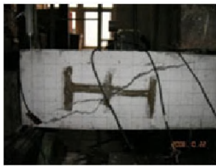
Figure 12 Shear failure of RC
