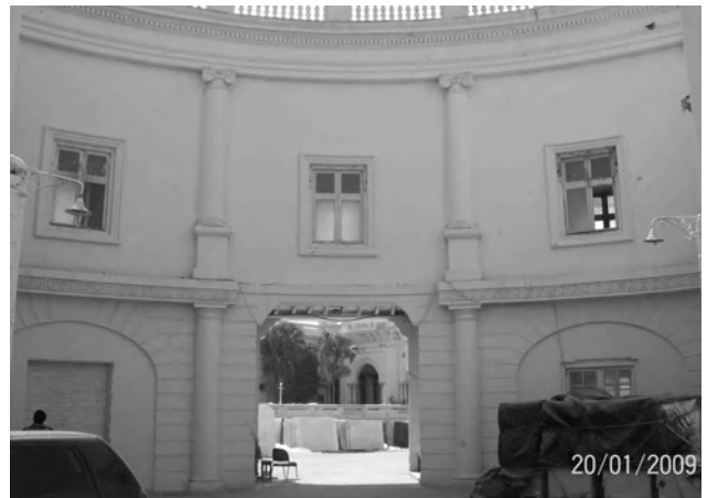
Figure 2 A wall panel at site identified for structural remediation
