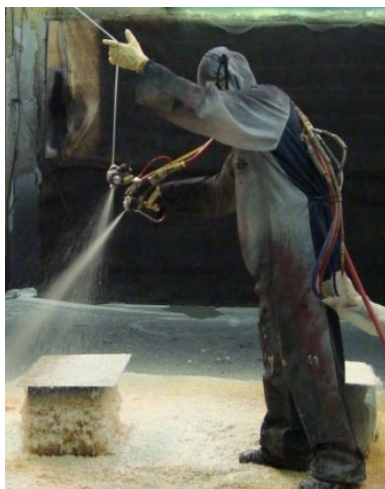
Figure 1 Polyurea application process
