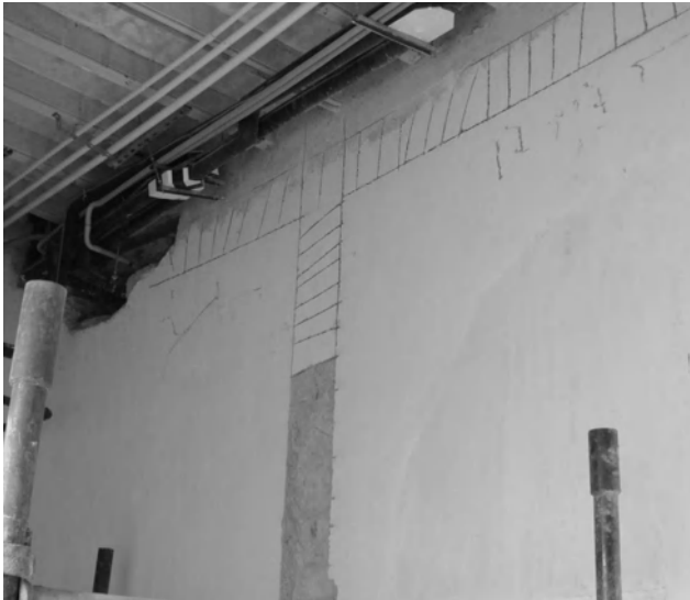
Figure 4 Marking of CFRP strip locations and removal of lime mortar rendering
