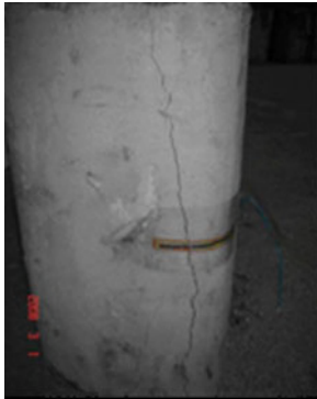
Figure 7 Failure mode for original specimen
