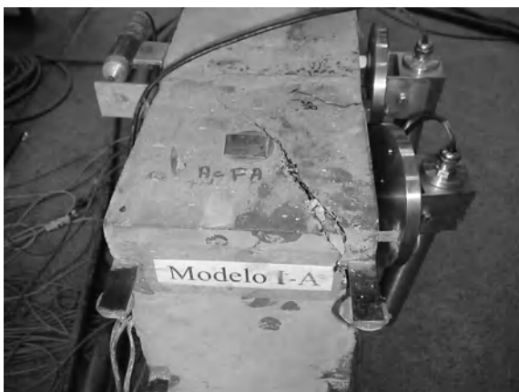
Figure 4 Connection region after failure
