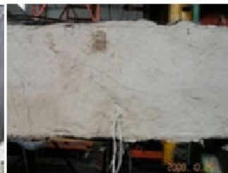
Figure 15 Shear failure of FRP GRID&ECC-RC
