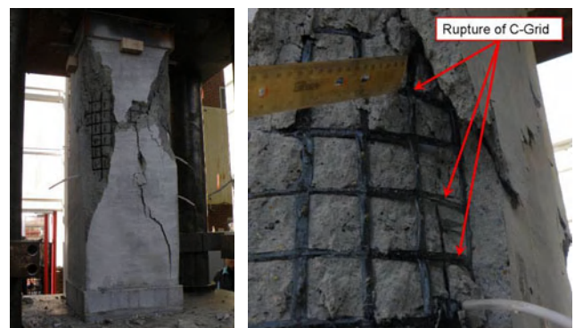
Figure 2 Column 2C-C-8 at the conclusion of the test
