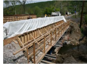
Figure 7 Formwork for concrete repair
