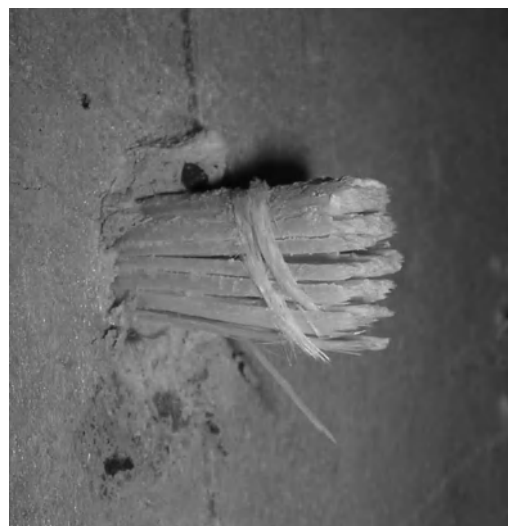
Figure 4 Failure of GFRP connectors
