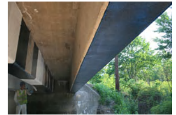
Figure 8 FRP strip installation
