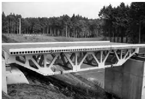
Figure 1 FRP truss bridge (in 2000)
