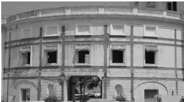
Figure 5 View of a wall panel with prepared surface ready to receive CFRP strips
