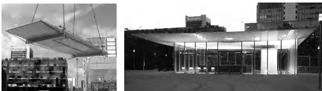
Figure 2 Multifunctional GFRP sandwich roof of Novartis Campus Main Entrance Building, 2006
