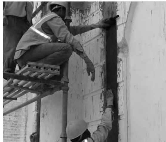
Figure 6 Installing vertical CFRP strip onto a wall panel
