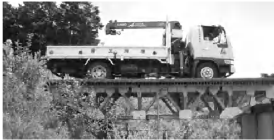
Figure 2 Loading test (5-ton, 2009)
