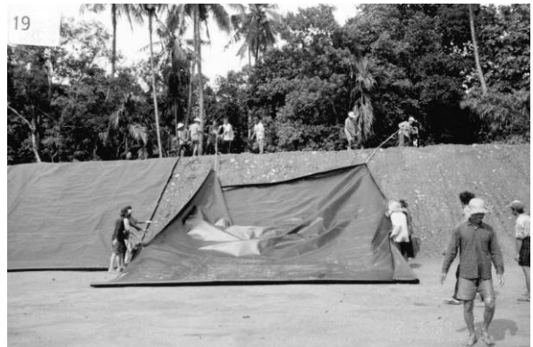
Fig. 6 Geomembrane deployment
