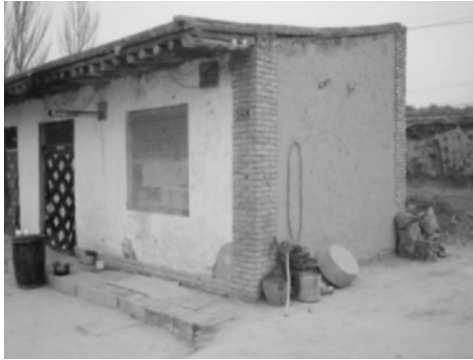
Fig. 11 A Brickcolumn load-bearing building
