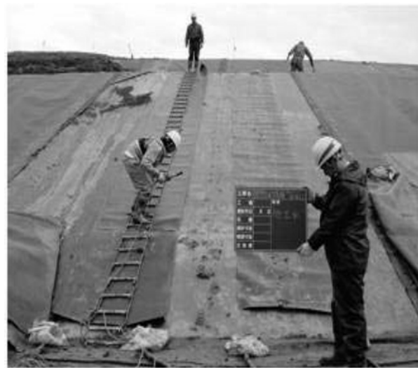
Fig. 52 Sheet installation condition
