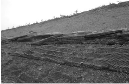
Fig. 5 Implementation of flexible supporting for ramp slopes
