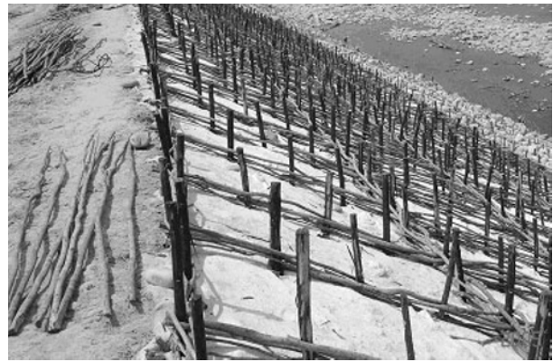
Fig. 16 Ryushikou revetment under Construction
