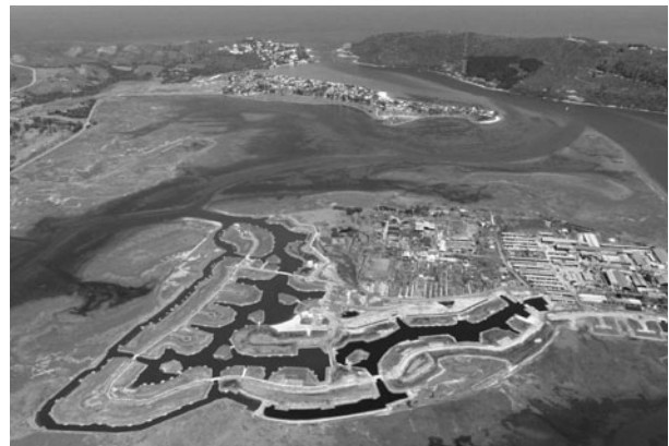
Fig. 9 Aerial view of Thesen Islands
