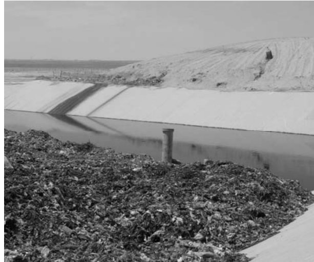
Fig. 1 Leachate generated from biodegradation of organic waste at a landfill site located in a desert. Note black and brown leachate stain due the leachate leaking from the adjacent completed cell (upper left) into the operating cell (foreground)
