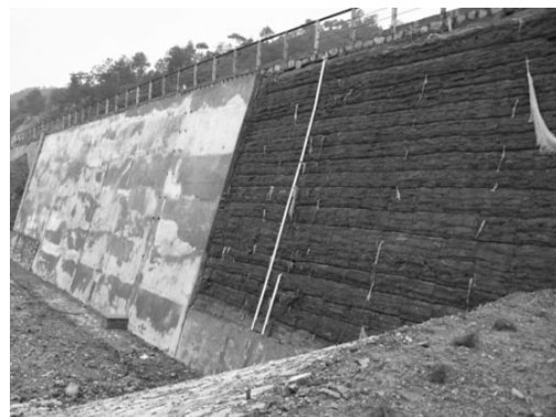
Fig. 1 Photo of the geogrid reinforced soil retaining wall with wrap-around facing
