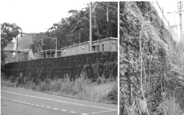
Fig. 3 Gabion retaining wall
