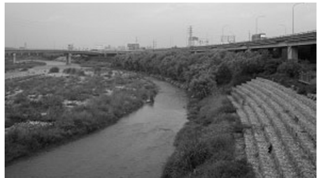
Fig. 17 Current condition of the embankment with box gabion and Ryushikou Revetments along the river
