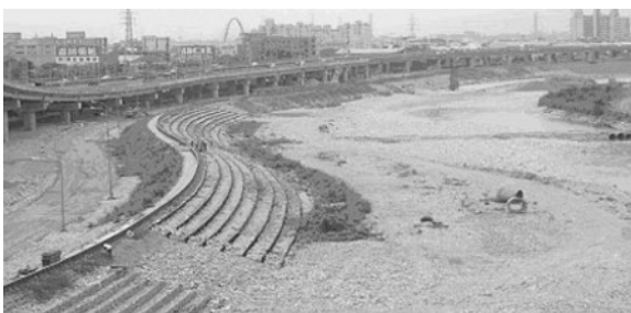
Fig. 15 Stairs-like revetment under construction
