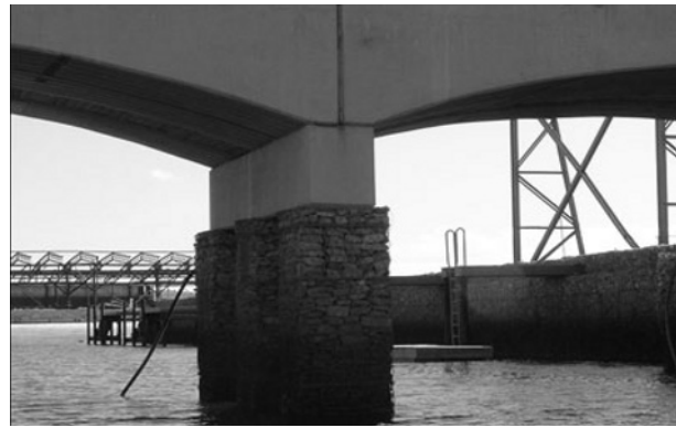
Fig. 8 Gabion bridge pier protection
