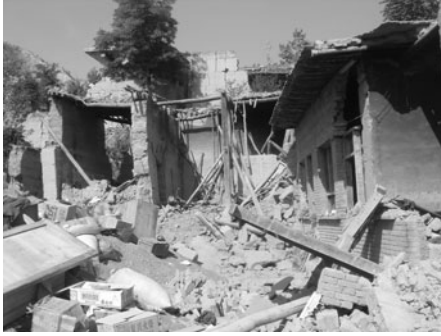
Fig. 6 Damages of adobe-wood building in Yingzhuang Village of Xihe-County(VIII degree area)
