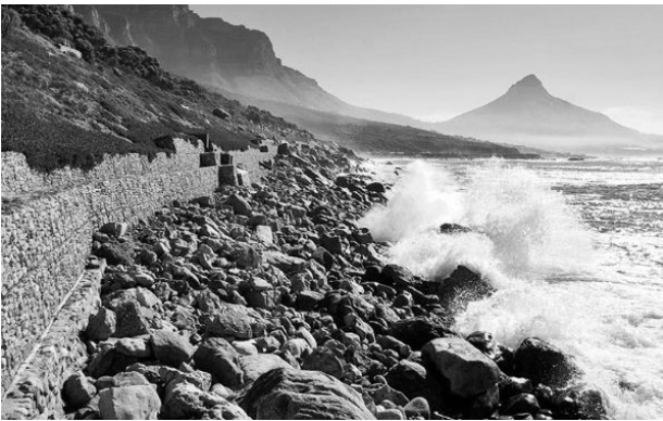
Fig. 10 Gabion coastal protection
