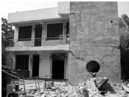
Fig. 1 A brick-concrete building at Bikou Village, Wenxian County, Gansu Province. (IX degree)
