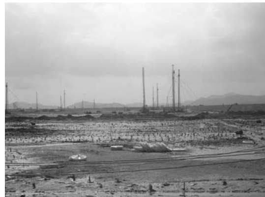
Fig. 6 Overview of the in-situ test at Lingang Industrial Zone, Tianjin, China
