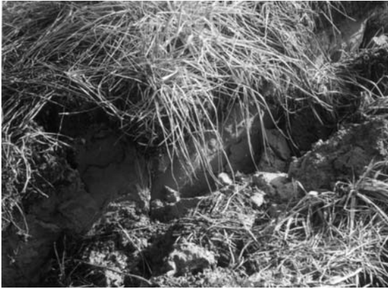
Fig. 15 Cracks widening between sliding blocks
