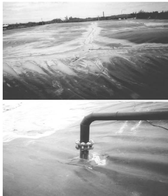
Fig. 3 Storm water weight pipe (Top) and connection pipe from the excretion pond (Down)
