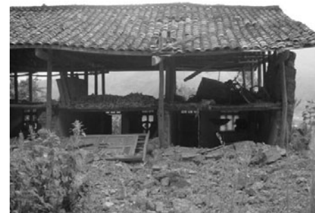
Fig. 4 A wood-frame house was damaged seriously at Kongjiashan Village, Wenxian County, Gansu Province. (IX degree area)
