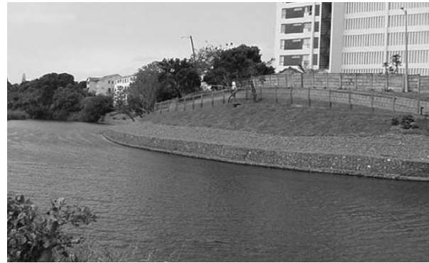
Fig. 4 Gabion & reno mattress longitudinal structure
