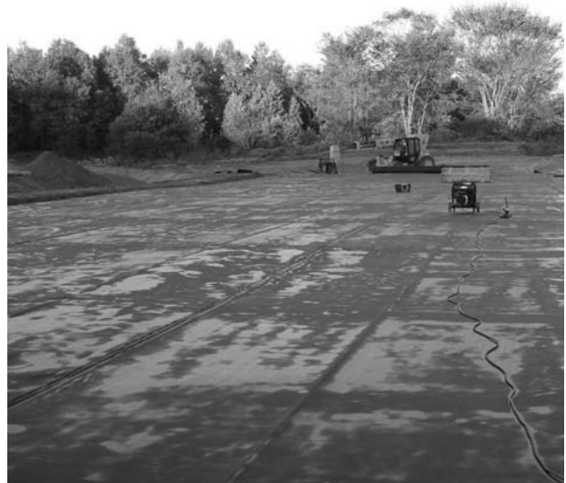
Fig. 2 Geomembrane placed without any significant wrinkles at Queen's Experimental Liner Test Site, Godfrey Ontario. Geomembrane and clay are in direct contact. Note the almost imperceptible crease line (due to blown film process) in the middle of the photo. A similar crease line is shown later in the day (after thermal expansion of the geomembrane) in Fig. 3
