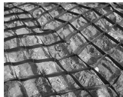
(a) Construction (spreading geocell)
