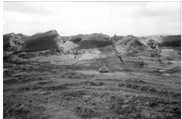
Fig. 4 Landfill Waste Stability Failure
