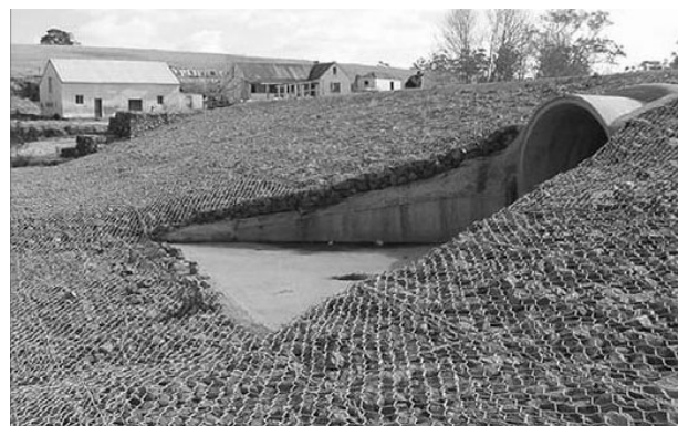
Fig. 6 Reno mattress culvert
