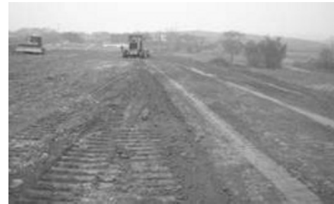
Fig. 2 Construction of expansive soil embankment by the enveloping method
