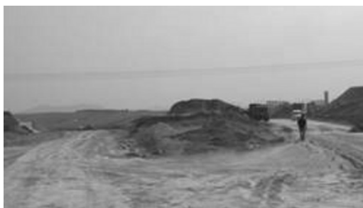
Fig. 3 Partly excavation of center-island
