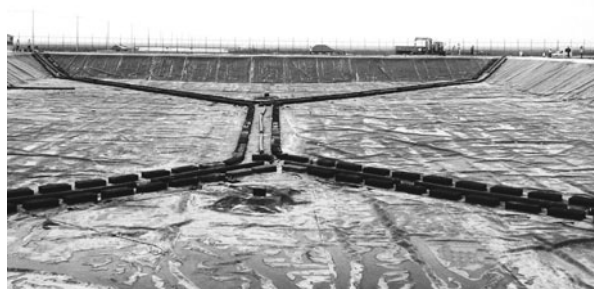
Fig. 4 A Completed HDPE Geomembrane Floating Cover System in Shanghai, China
