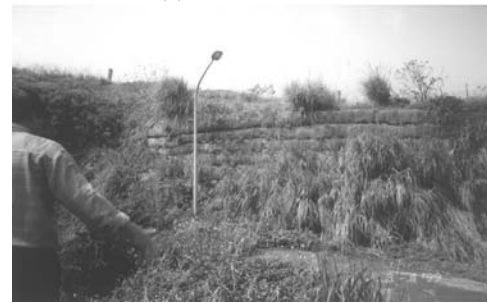
(b) Reinforced retaining wall at the toe of slope
