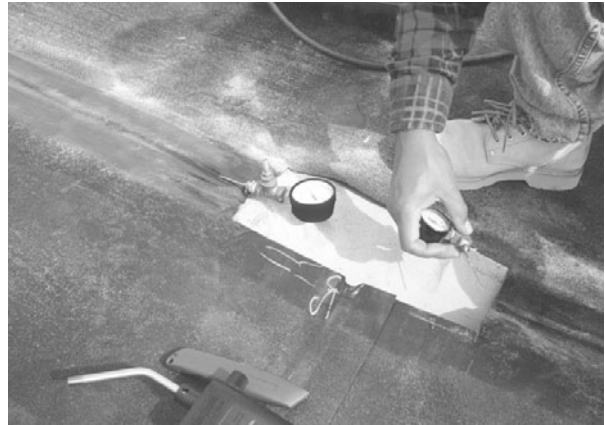
Fig. 5 A Non-destructive air pressure test is in progress.
