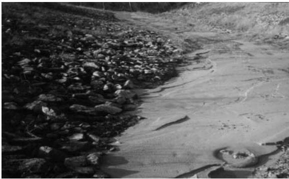
Fig. 16 Vegetative support soils washed to slope base
