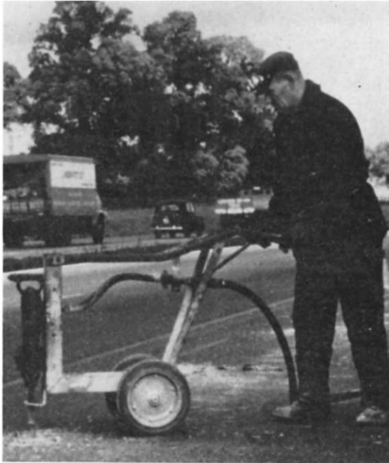
FIG. 74. A pneumatic tool for breaking out defective concrete prior to repair.
