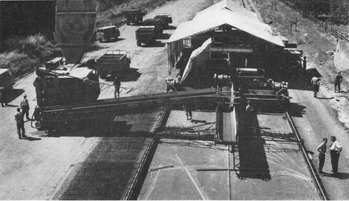
FIG. 27. A travelling paver mixer feeding a spreader by moving belts on a large-scale motorway contract. Note (1) lorries bringing dry batched concrete for mixer, (2) reinforcement laid ready for placing, (3) plastic film laid on base, (4) tents covering spreading and finishing machines for protection from the weather.
