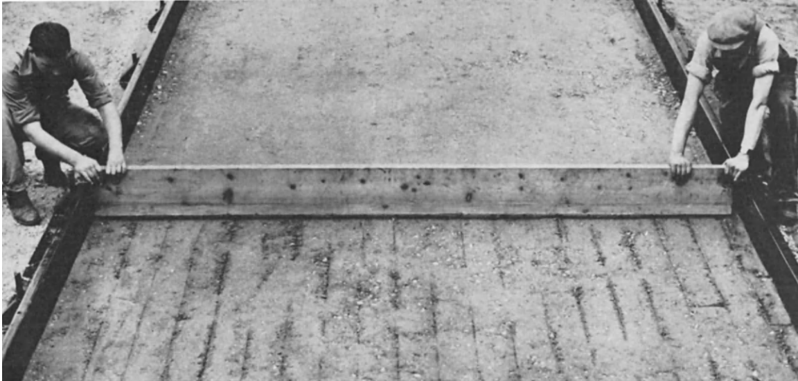
FIG. 15. Checking the accuracy of the sub-base with a scratch template, using the forms as a datum.
