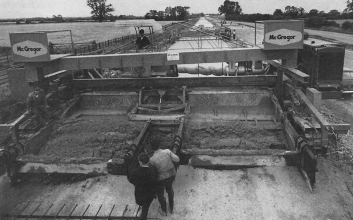
FIG. 44. Concrete tipped into the front of a slip form paver.
