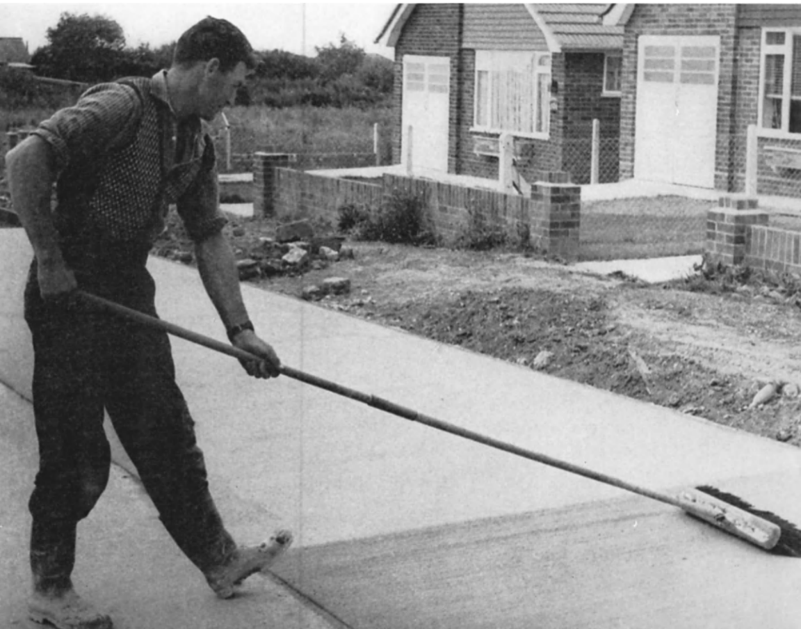
FIG. 19. Forming a lightly brushed texture on a housing estate concrete road.
