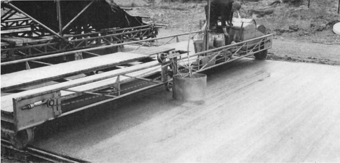
FIG. 40. A self-propelled automatic membrane curing compound sprayer.
