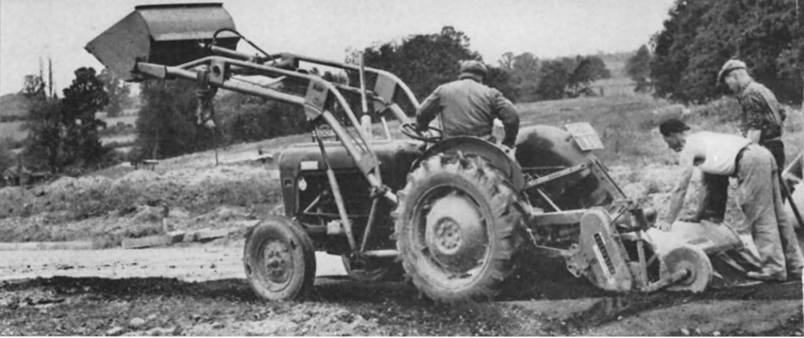
FIG. 46. A 4-ft-wide offset multi-pass mixing machine fitted to a standard tractor.
