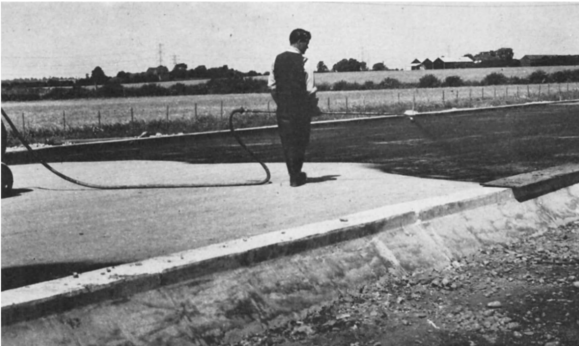
FIG. 56. Bituminous emulsion being sprayed on a lean concrete base for curing.
