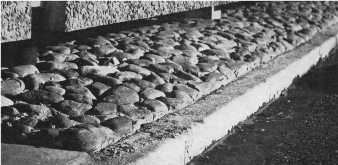
FIG. 89. Precast concrete exposed aggregate panels used to face a dividing strip on a central reservation. The cobblestones are set in concrete.
