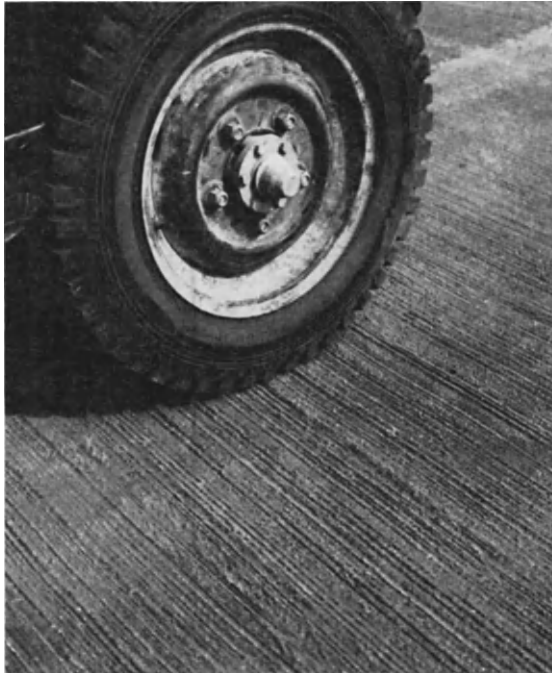
FIG. 75. A typical brushed texture with an average texture depth of about 0.30 in. for high-speed roads.
