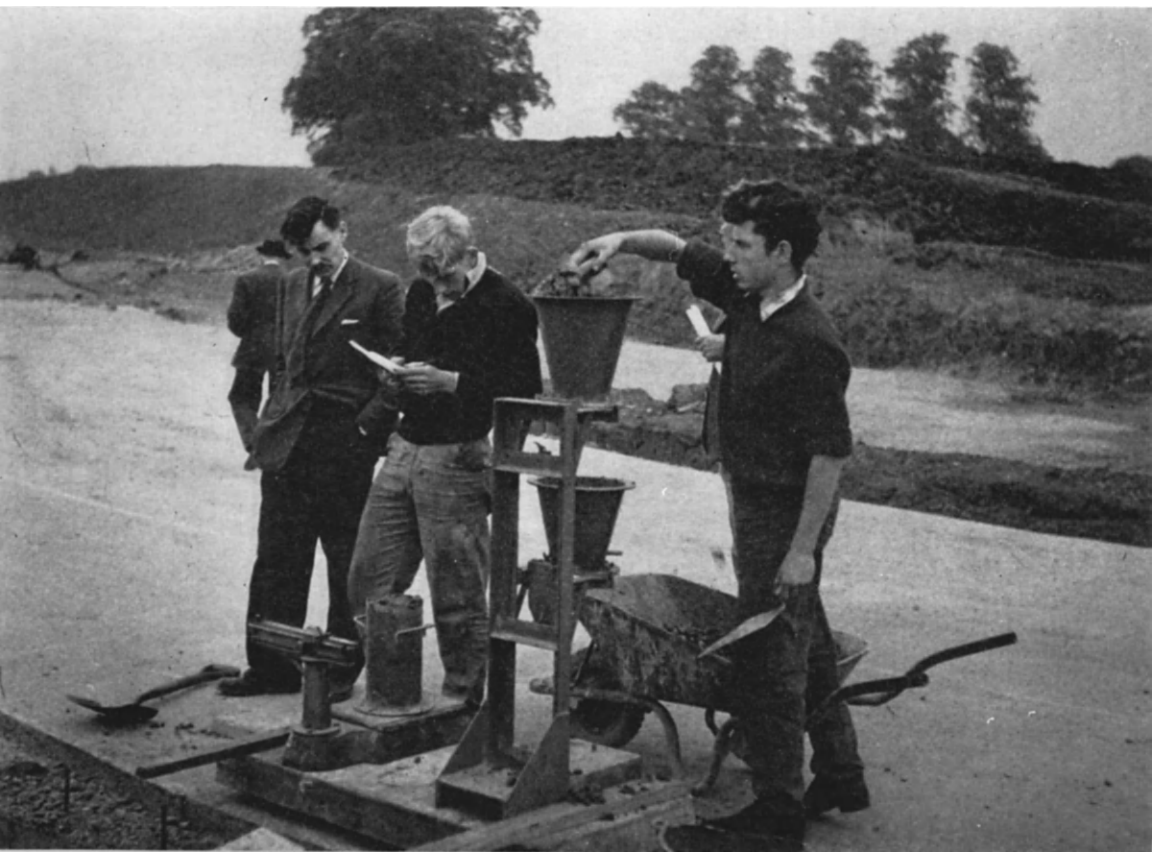
FIG. 1. The compacting factor test being used on a site to determine the workability of the concrete.
