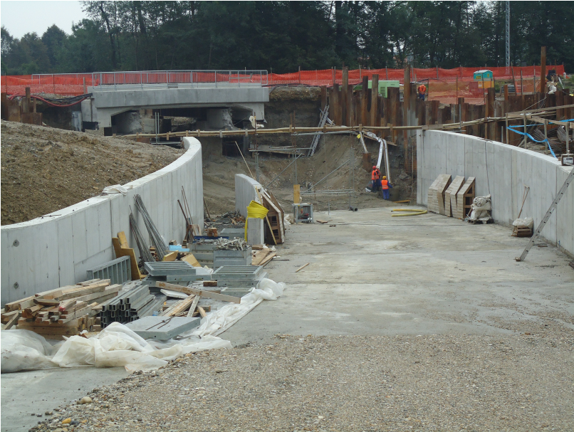
Fig. 5. Construction site “Underpass Grlava”: use case for application of knowledge model
