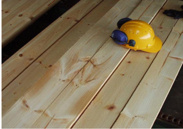
Fig. 9.13 Compression wood formed around knots and a previously damaged leader in Sitka spruce (photograph B. Gardiner)
