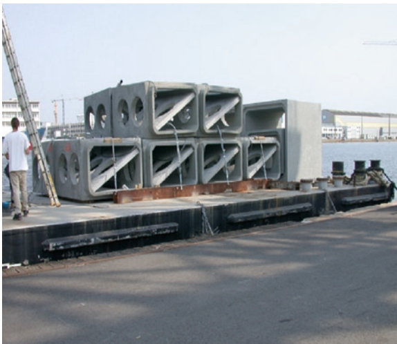
Fig. 2 Organized assemblages of reefs before their immersion
