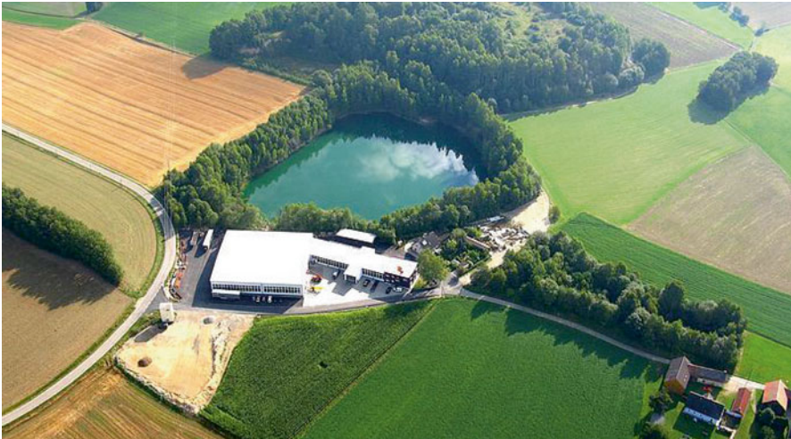
Fig. 1.4b Oblique aerial view of the flooded open pit with the overburden and dumps in the background at Hagendorf-South already covered with a slash green vegetation of hardwood trees and shrubs. The mining area has been reclaimed and reused by a metal-working company while the mining relics have been converted into a nature-sanctuary. Sampling is no longer an easy task
