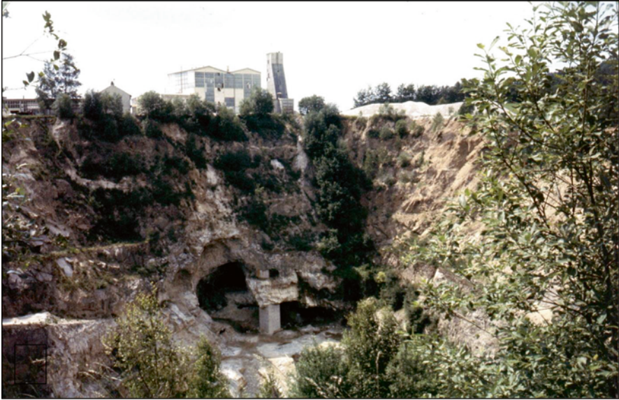
Fig. 1.4a Immediately after mining ceased in 1982, the open pit has not yet been flooded and still allows a look at the underground works with the mined out chambers and pillars stabilizing the roof. The mining edifice with the head frame of the inclined shaft still visible on the western edge of the open pit (Courtesy of G. Rank)
