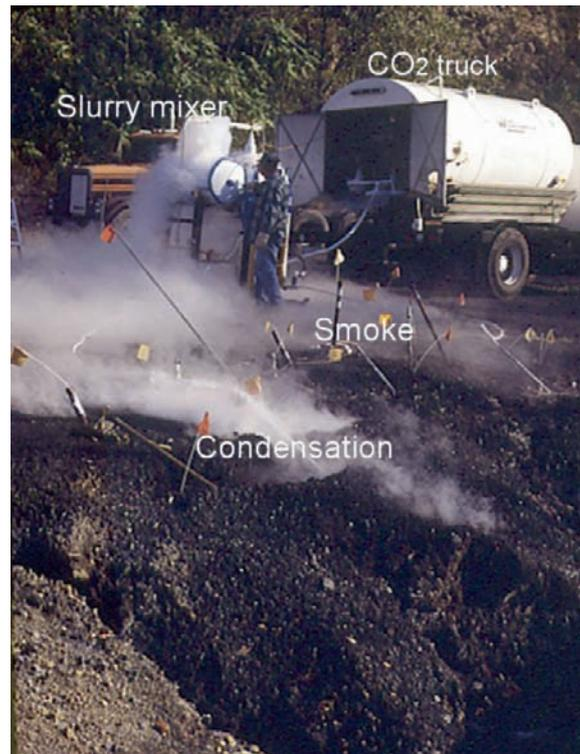
**Figure 16.5.6.** Photo of injection of cryogenic slurry at Midvale waste bank showing CO<sub>2</sub> truck, slurry mixing tank, emission of smoke from the bank, and condensation above the bank.
