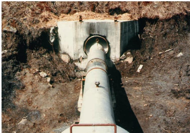
**Figure 16.5.3.** Photograph of a combustion manifold and a steel liner inserted into the Albright waste bank. From Chaiken and Bayles 1991, p. 10.
