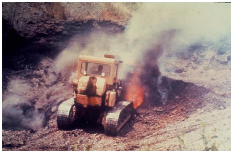
**Figure 1.2.5.** Excavation involves the hazards of working in hot material and toxic fumes. US Bureau of Mines photo 1982, Calamity Hollow Burnout Control Project.
