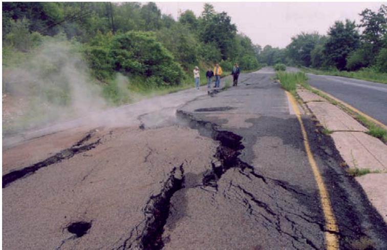
**Figure 7.1.6.** Route 61 through Centralia, PA. The cracks are due to subsidence of the road into abandoned coal-mine tunnels beneath the road. Subsidence occurs when coal pillars supporting the roof of a tunnel burn and collapse. Note the toxic gas exhaled along the cracks. Photo by Janet L. Stracher, 2003.
