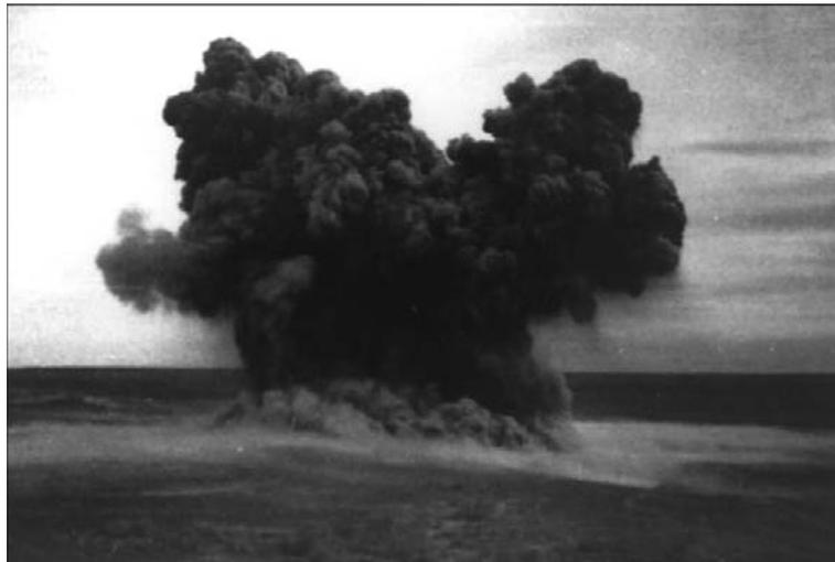
**Figure 5.1.3.** Controlled-directional blasting used to extinguish an underground coal-mine fire, Beishan coalfield, Qitai County, China. Reproduced with permission of Taylor & Francis. After Bell and Donnelly 2006; photo by Bell 1985.
