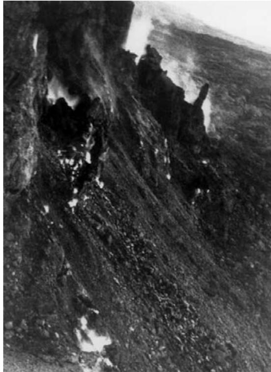
**Figure 5.1.10.** Coal seams burning in an opencast coal mine in the Beishan coalfield, Qitai County, China, resulting in toppling failure, sliding, and collapse downslope. Reproduced with permission of Taylor & Francis. From Bell and Donnelly 2006. Photo by Bell 1985.
