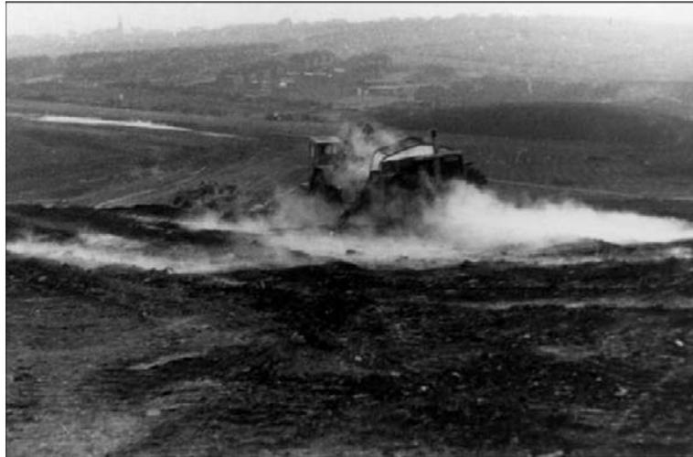
**Figure 5.1.12.** Leveling and reprofiling of a spoil heap undergoing spontaneous combustion, Barnsley, England. Photo by Bell 1985.
