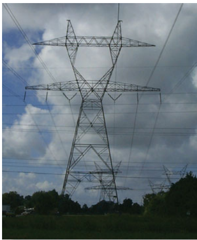
For economic reasons, large electrical transmission towers are often constructed using space trusses.
