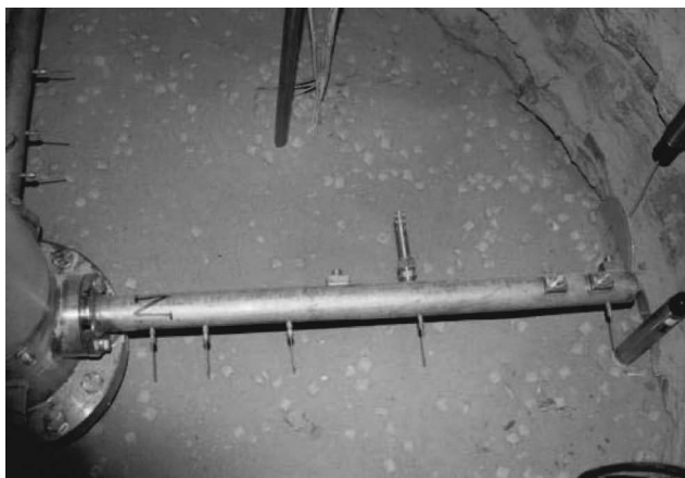
Fig. 1. Mixture of bentonite pellets and bentonite powder used as sealing material in an experimental shaft
