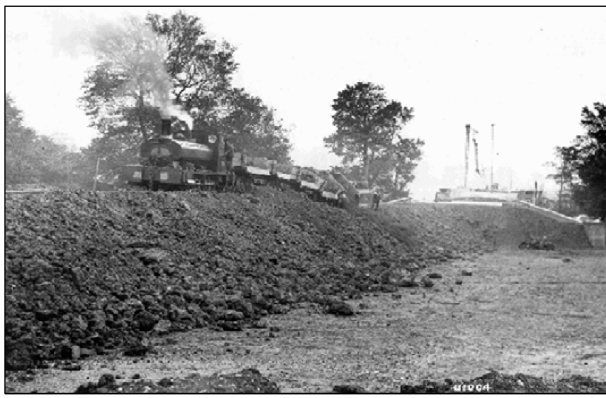
Embankment construction (a)
