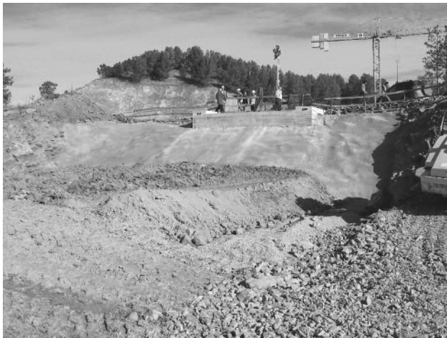
Fig. 2. Clay core, filter and rockfill shoulder of Lechago dam during construction
