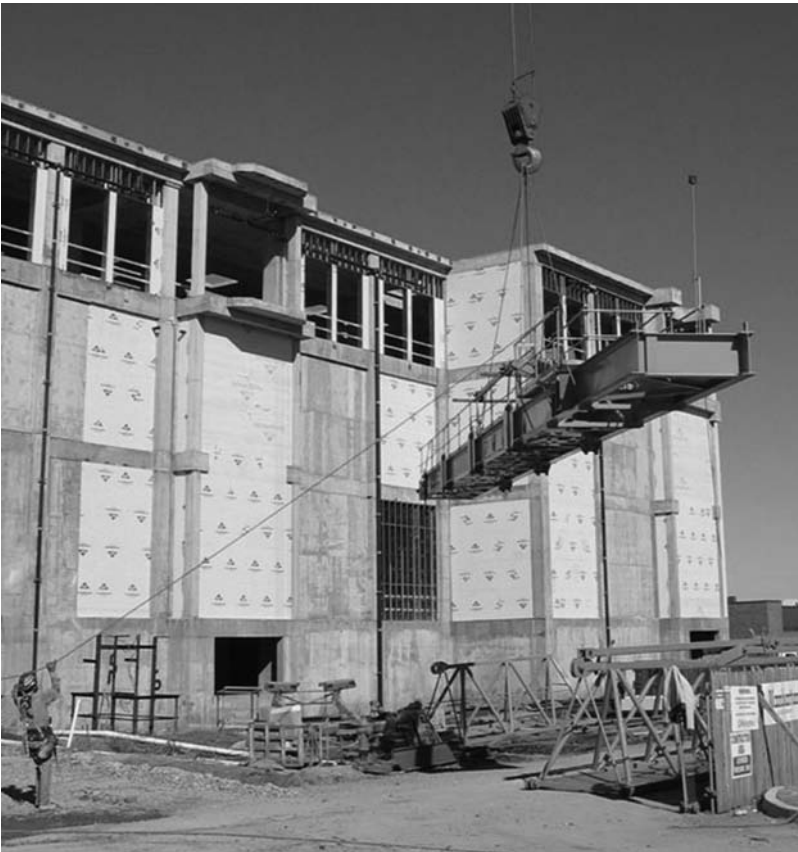
FIGURE 8.22 Lowering the counterdeck.
