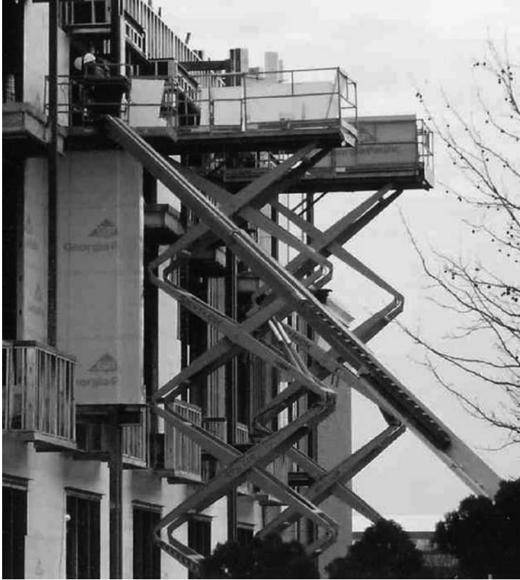
FIGURE 4.32 Scissor and telescoping boom personnel lifts.
