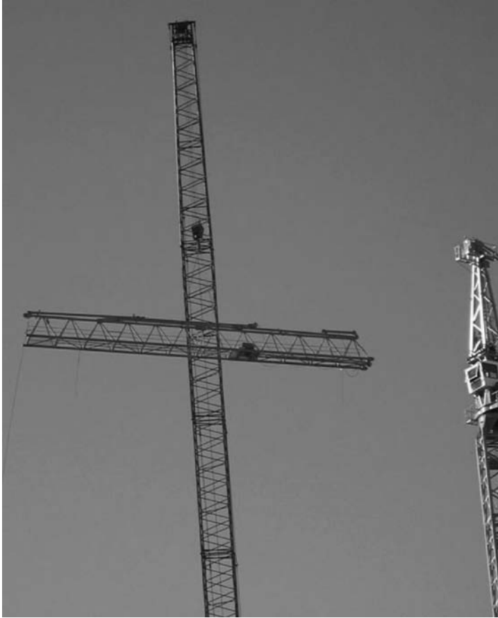
FIGURE 8.18 Disconnecting the remaining jib.
