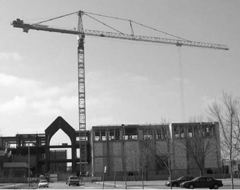
FIGURE 8.12 Horizontal jib tower crane.
