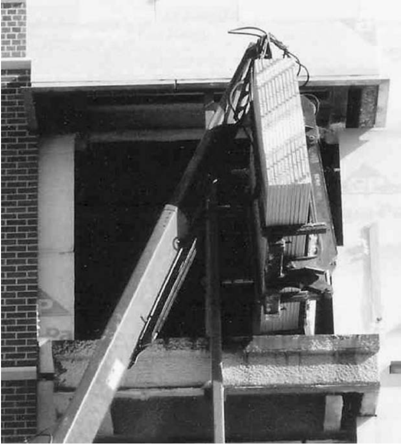
FIGURE 4.25 Sheetrock attachment.
