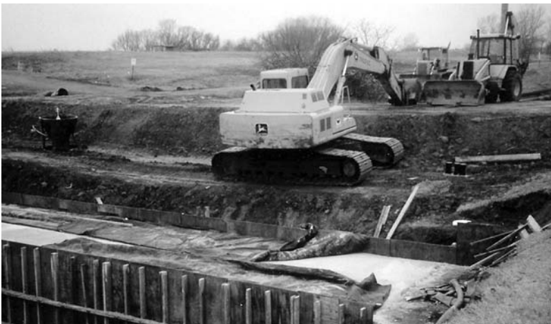
FIGURE 4.7 Excavator on a bench.
