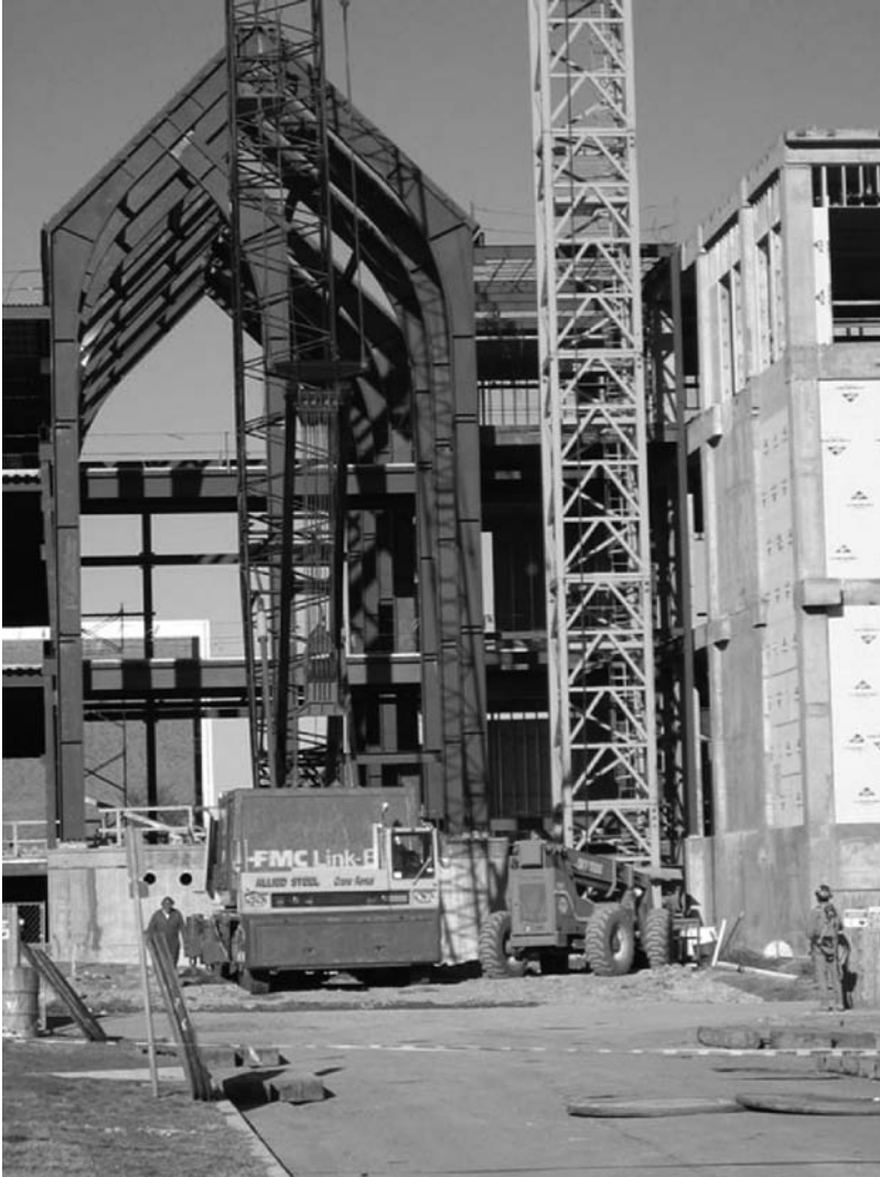
FIGURE 8.16 Support crane move.
