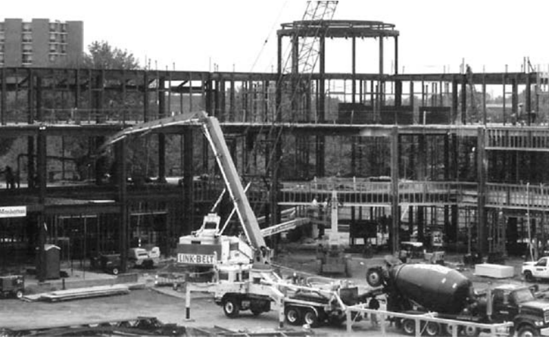
FIGURE 8.5 Pumping elevated flatwork.
