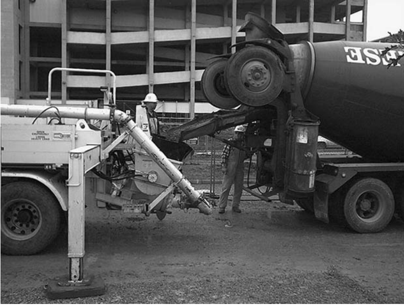
FIGURE 8.3 Chuting concrete into the pump hopper.
