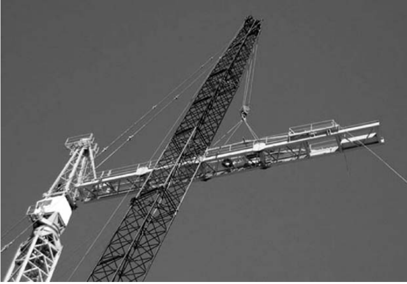
FIGURE 8.21 Dismantling the counterdeck.
