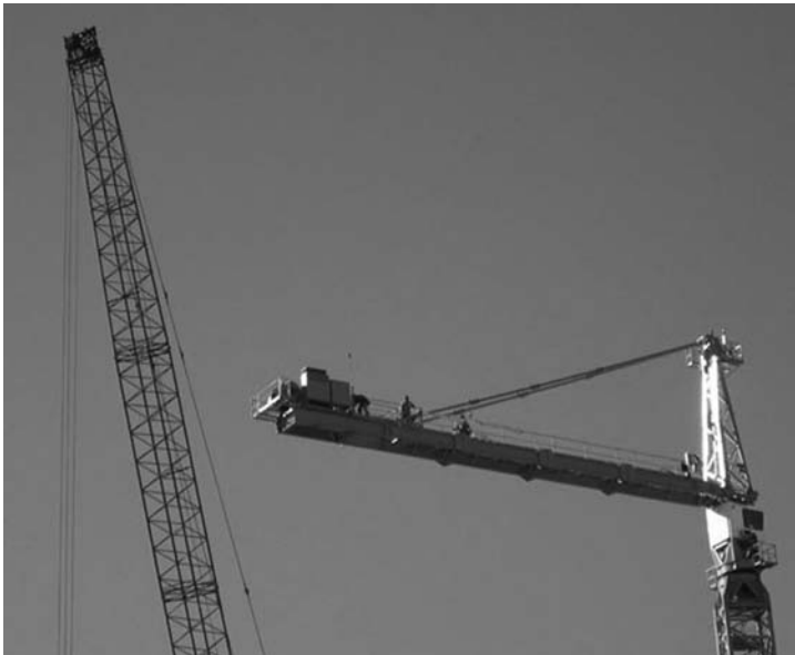
FIGURE 8.19 Positioning the counterdeck.
