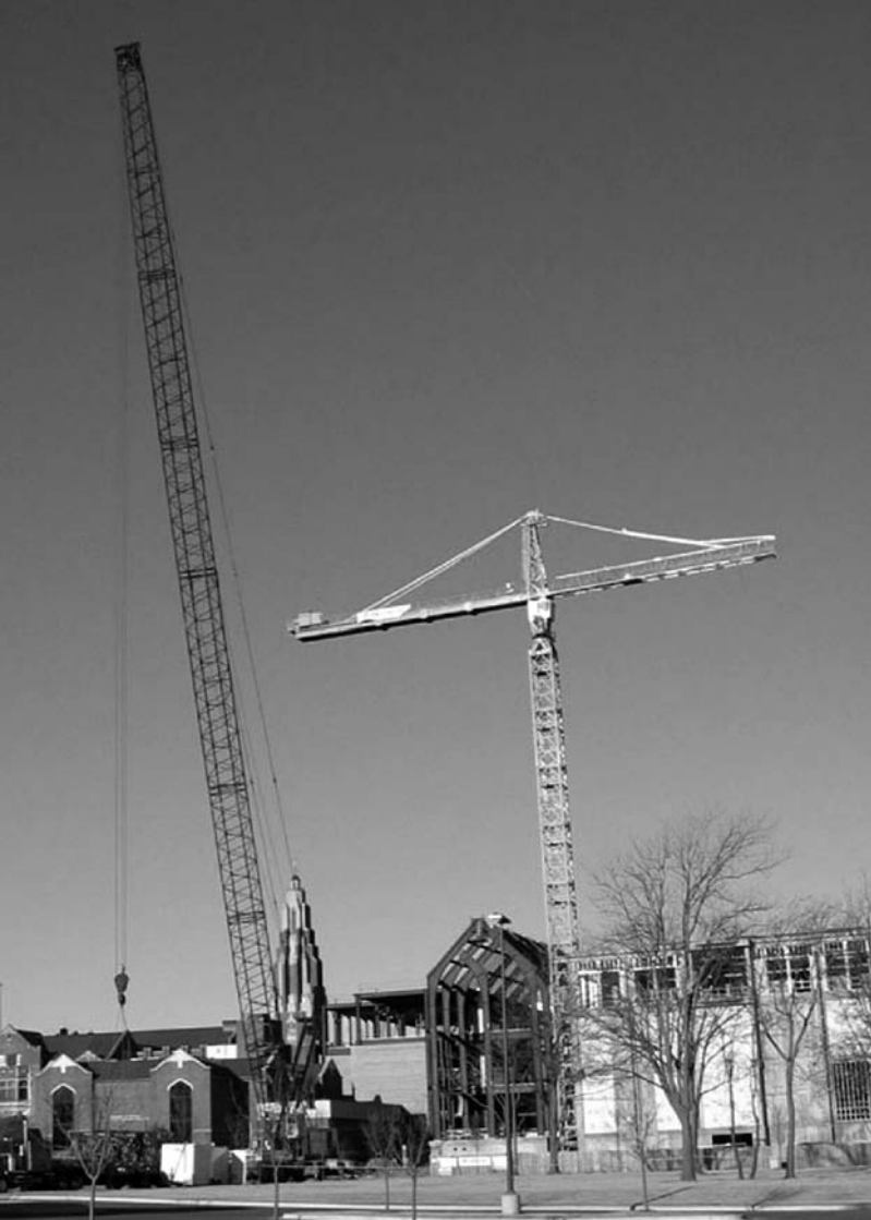
FIGURE 8.15 Two jib sections dismantled.
