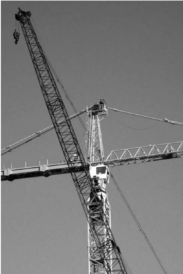
FIGURE 8.17 Riggers on the crane.
