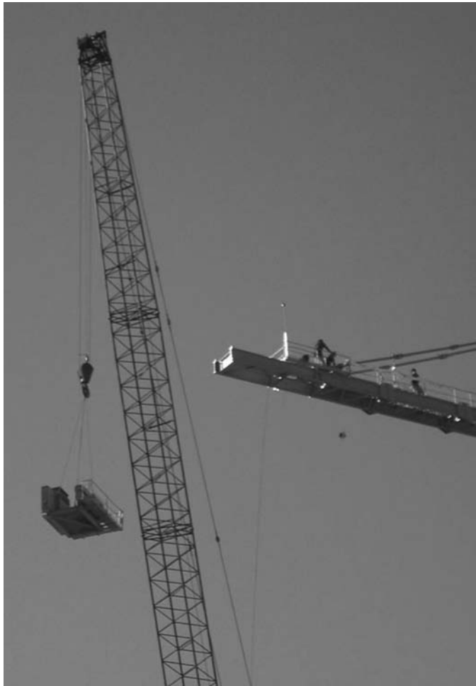
FIGURE 8.20 Removing the motor.
