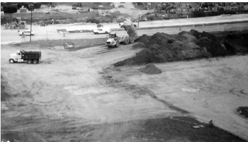
FIGURE 11.4 North side of site.
