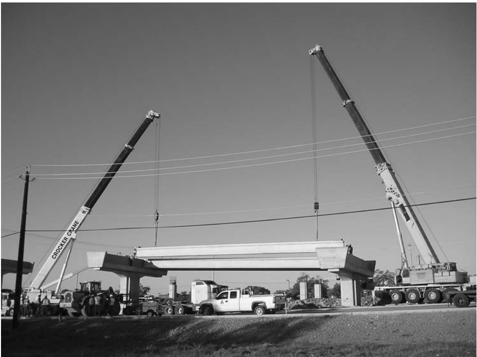
FIGURE 8.1 Dual lifting.
