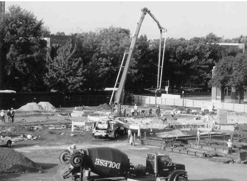
FIGURE 8.4 Pumping a slab on-grade.
