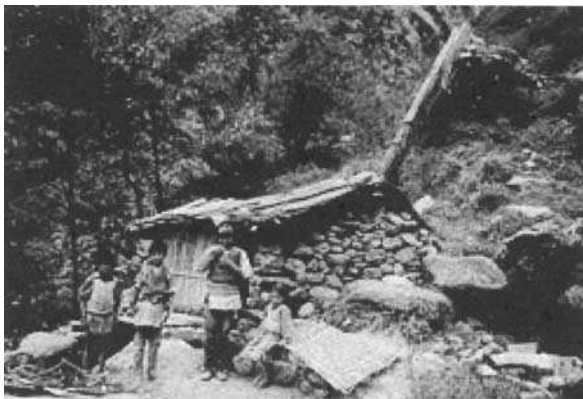
Figure D-1. Ghatta house (water mill)
