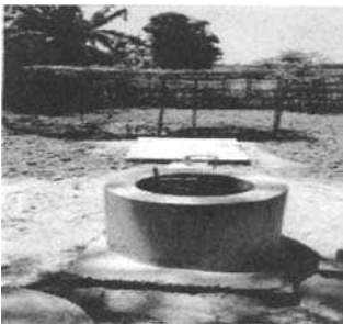
Figure A1. Biogas chamber
