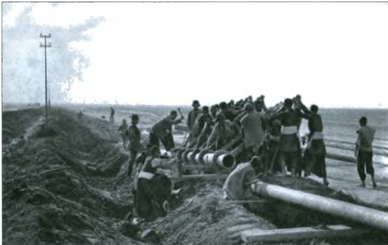
Laying pipe for the Anglo-Persian Oil Company, date unknown. (From: The Collection of the author. )
