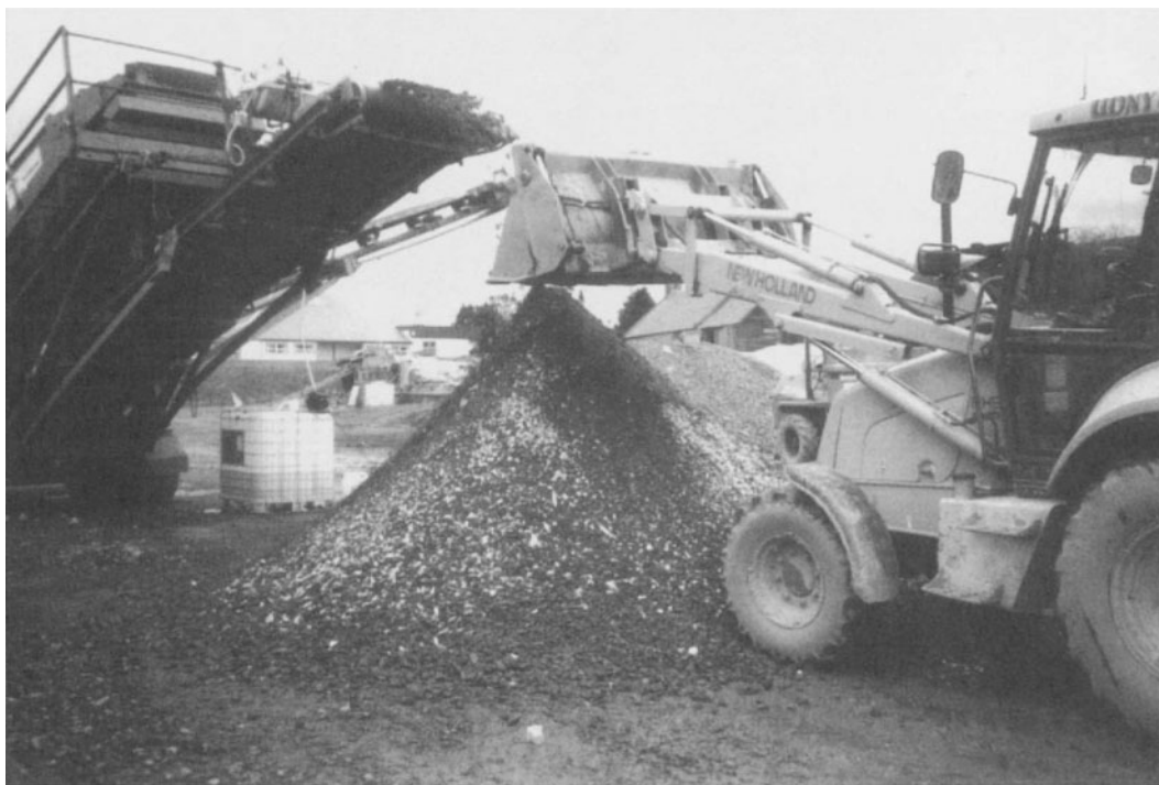
FIGURE 5.7 Photograph of soil screening and addition of wood chips (the lighter material in the soil heap) and bioaugmentation culture (contained in the 1-m 3 Intermediate Bulk Container), which is being applied by spray at the top of the soil grader.
