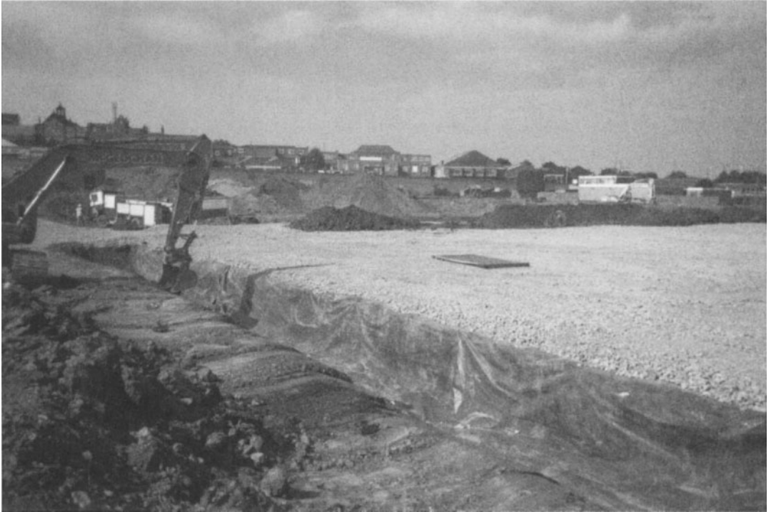
FIGURE 5.3 Photograph of a biopile base showing its preparation. Courtesy of WSP Remediation Ltd., Cardiff, United Kingdom.
